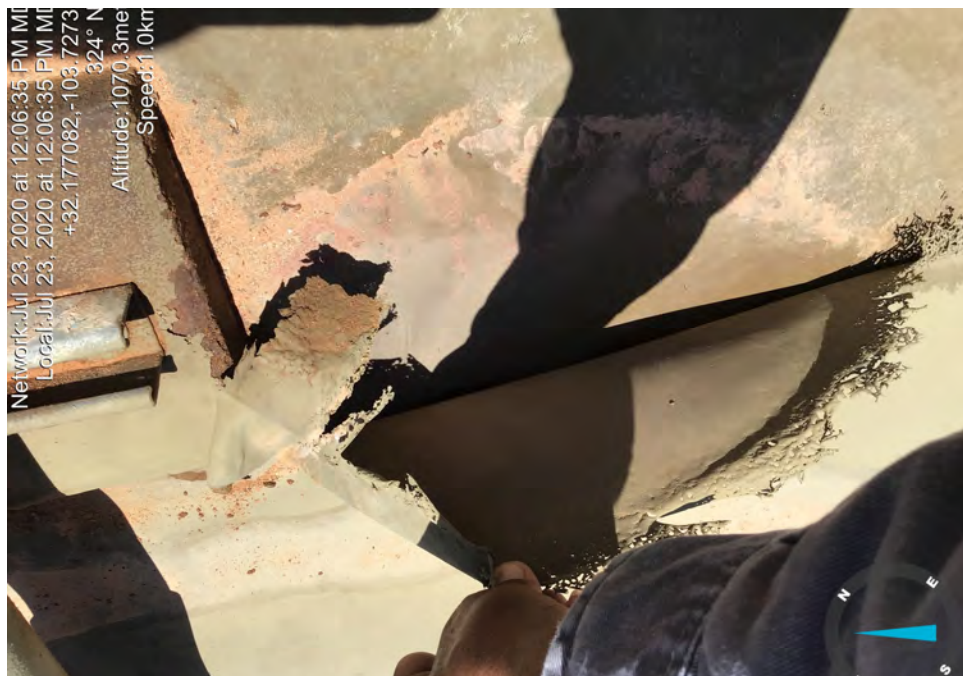
East side, inside pump#3, liner patch unglued
