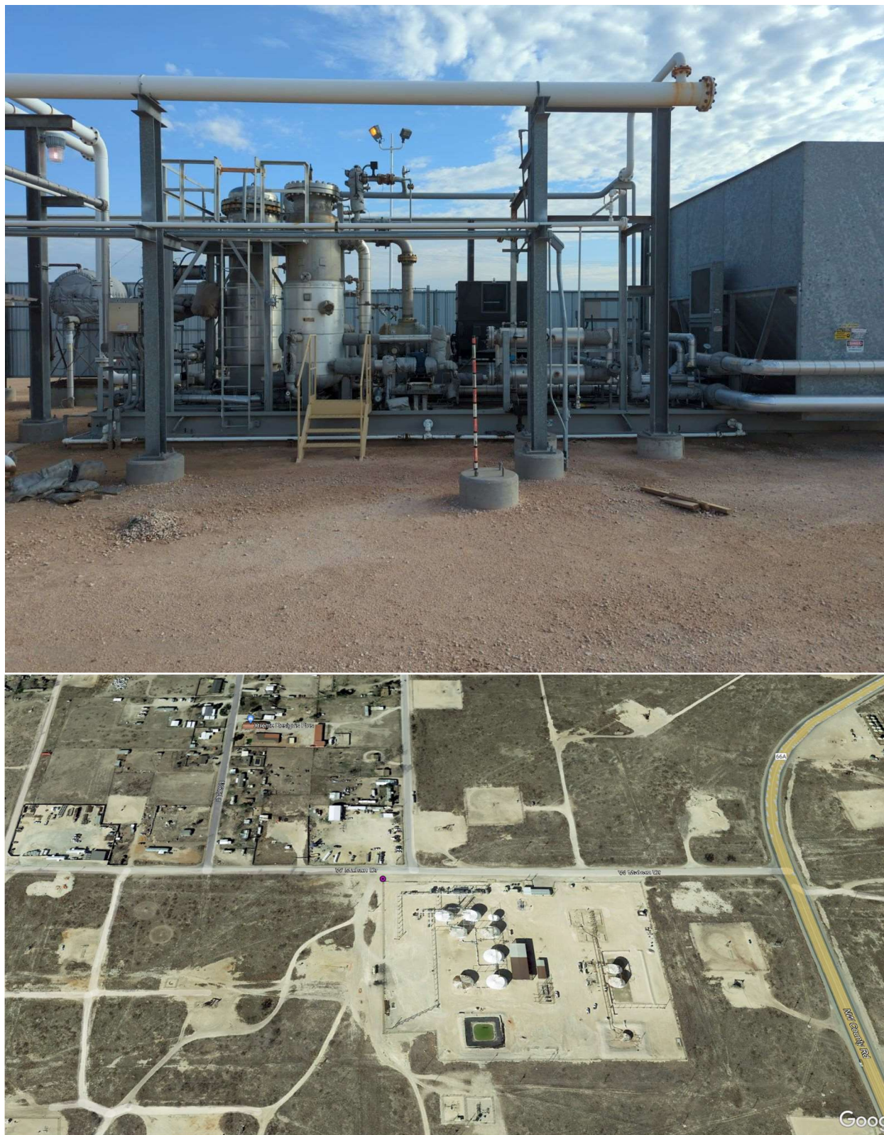
North Hobbs RCF lost train D compressor causing plant inlet pressure to spike and caused discharge pressure on the Toromont Compressor at the CTB to shut down on high high psi
