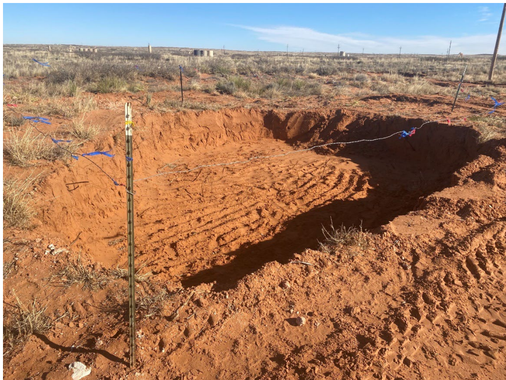
View of Area D excavation facing northeast.
