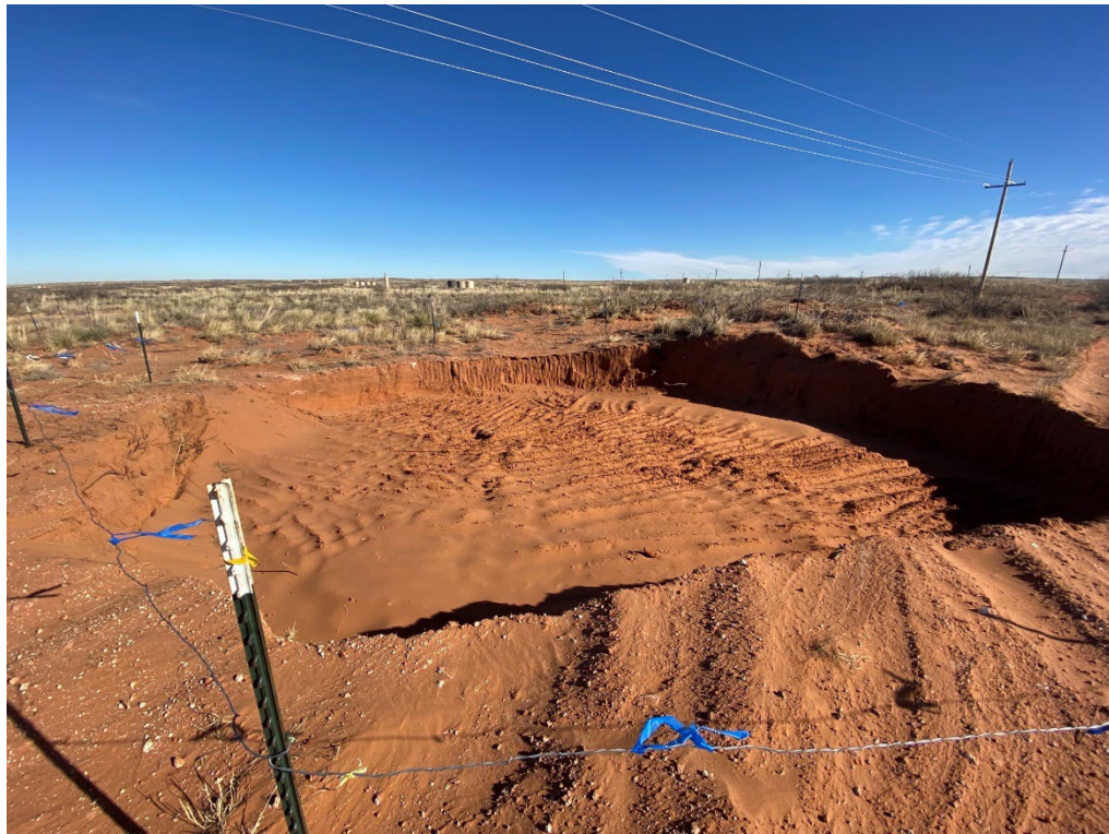
View of Area C excavation facing northeast.
