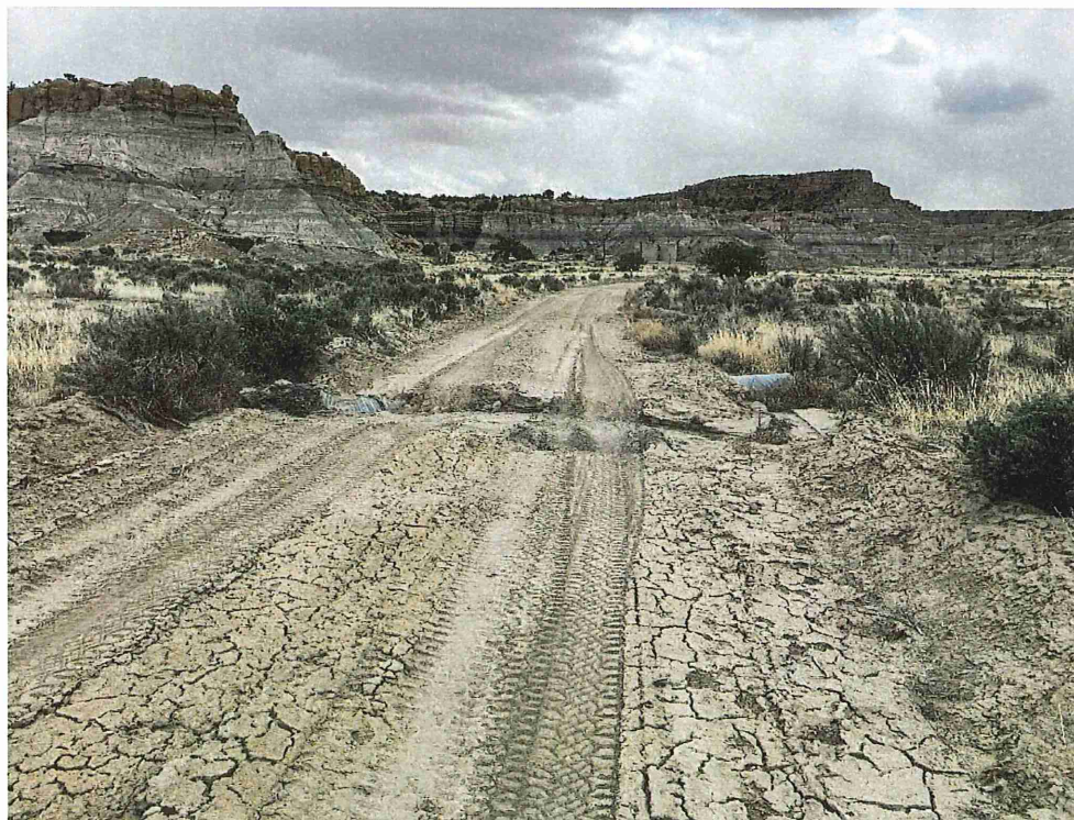
Photo 8: Access Road Erosion at Culvert
