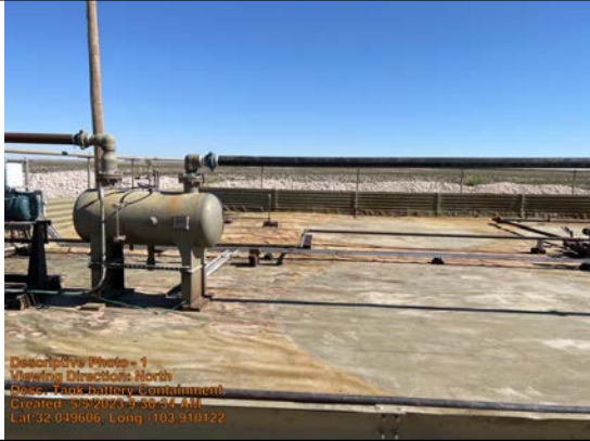
Tank battery Containment
