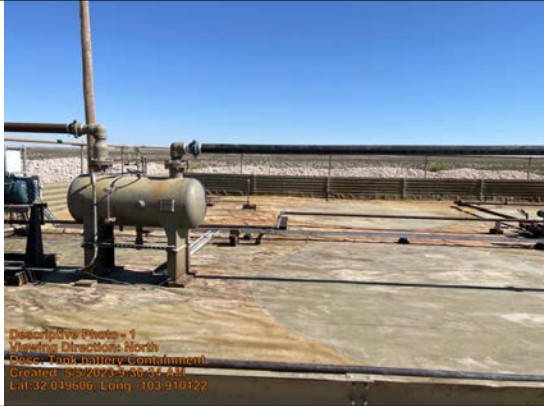
Tank battery Containment
