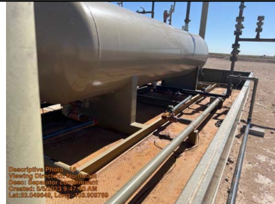
Separator containment
