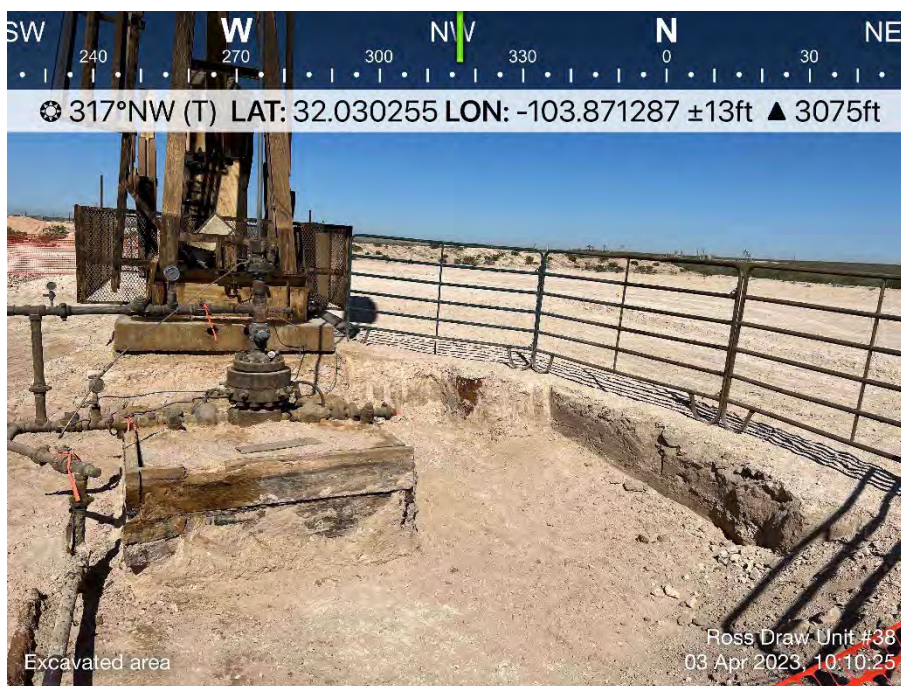
Excavated Area - Around Wellhead
