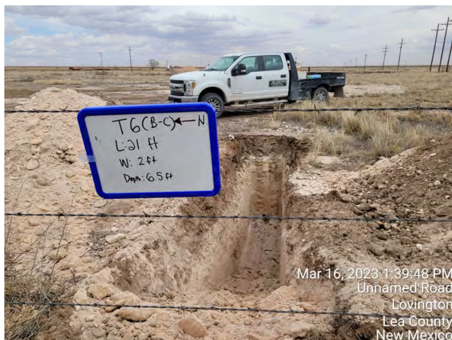
Photograph 13 — Trench excavation of T-6B through T-6C.
