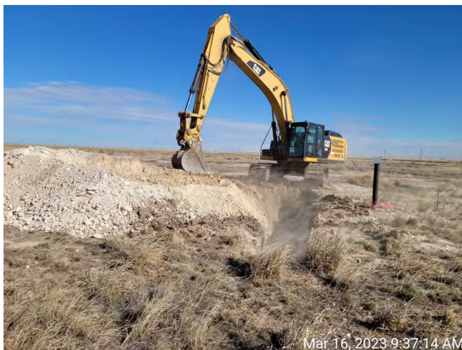
Photograph 22 -- Backfilling at T-5.
