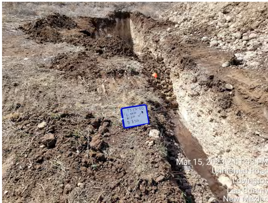
Photograph 9 -- Trench excavation of T-3A through T-3D.
