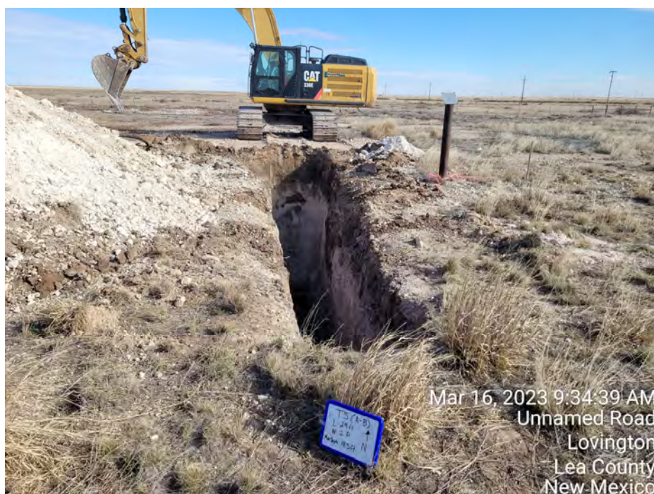
Photograph 11 — Trench excavation of T-5A through T-5B.
