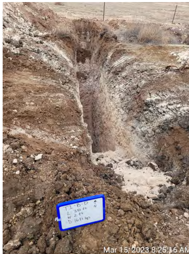
Photograph 8 -- Trench excavation of T-1B through T-1D.
