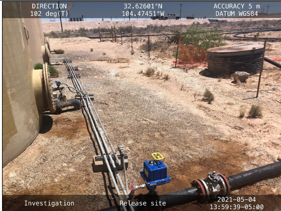
PHOTO 24: View of release point, facing southeast.
