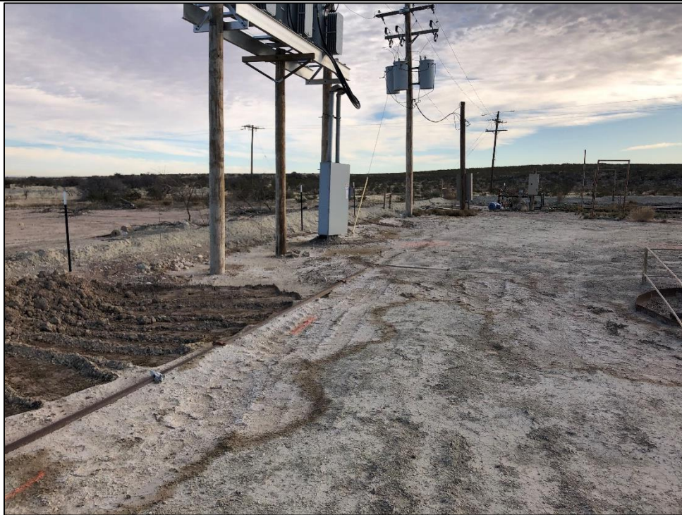
PHOTO 6: View of site, facing northeast. 11/22/2019 / TIME: 1:07PM / GPS: 32.1218 -1104.0725
