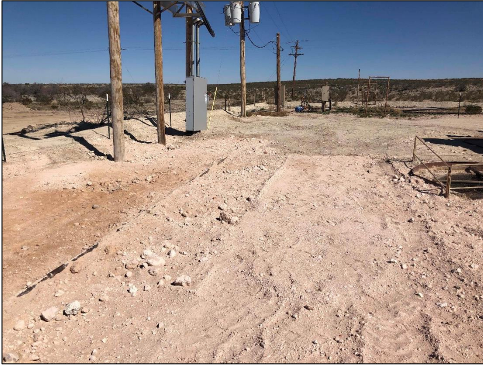
PHOTO 17: View of base of excavation, facing south. 11/22/2019 / TIME: 1:21PM / GPS: 32.1218 -1104.0725
