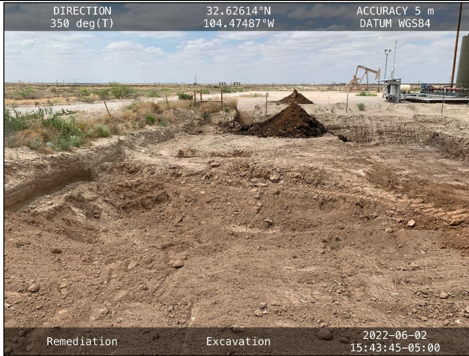
PHOTO 35: View of excavation in northwest corner, facing north.
