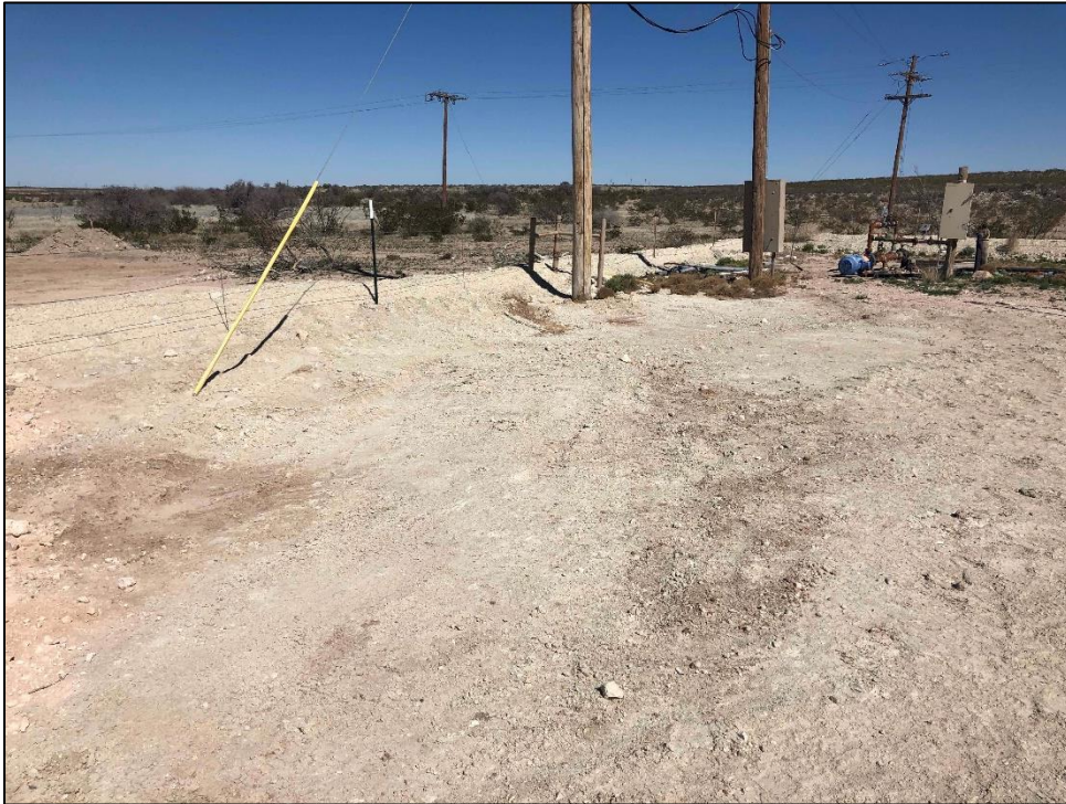
PHOTO 18: View of excavation, facing west. 11/22/2019 / TIME: 1:36PM / GPS: 32.1221 -1104.0725
