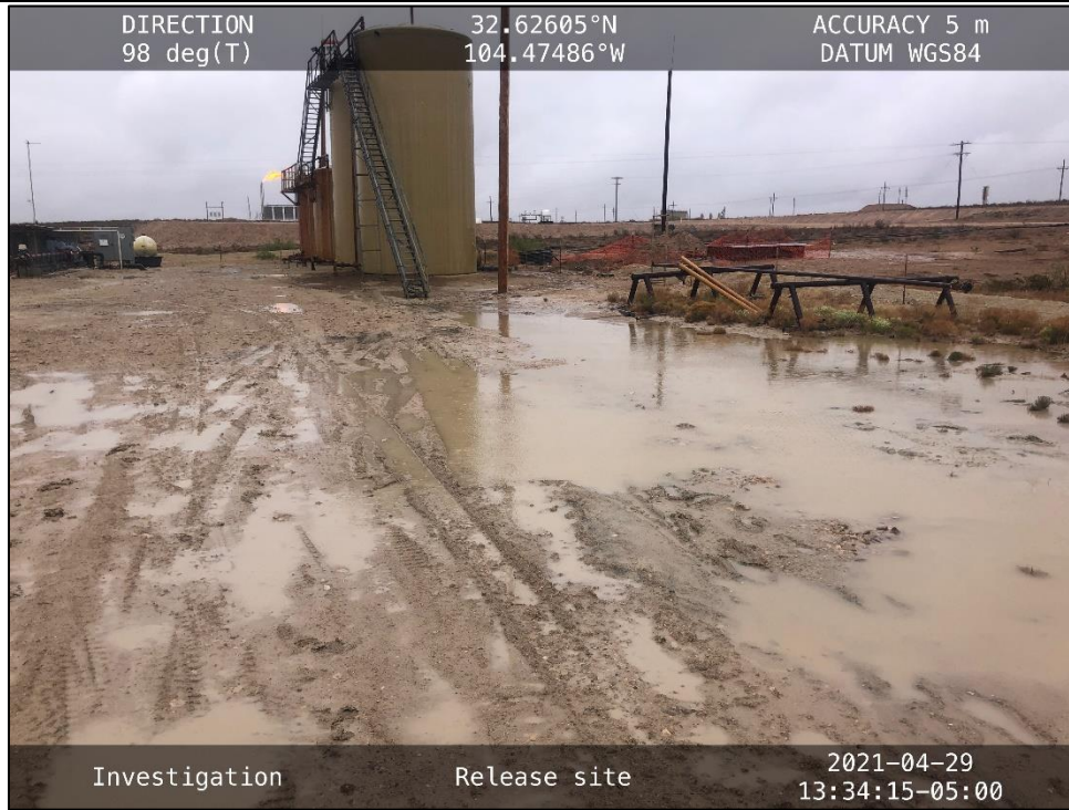
PHOTO 19: View of new release, facing east.
