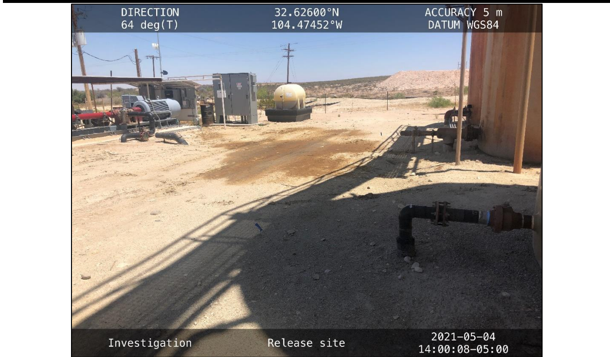
PHOTO 28: View of impacted soils, facing northeast.
