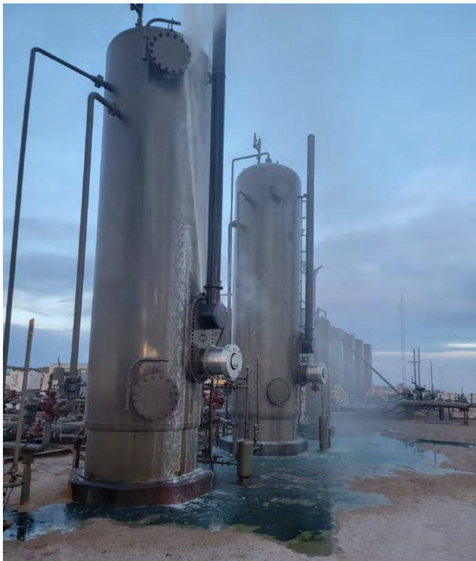
View northeast at heater treater and release from gasket, spill area
