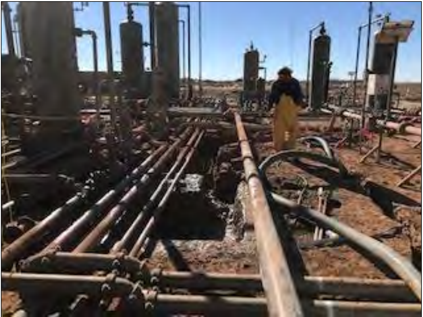
View south of excavation around surface lines within both release areas (2RP-4399 and 2RP-5026)
