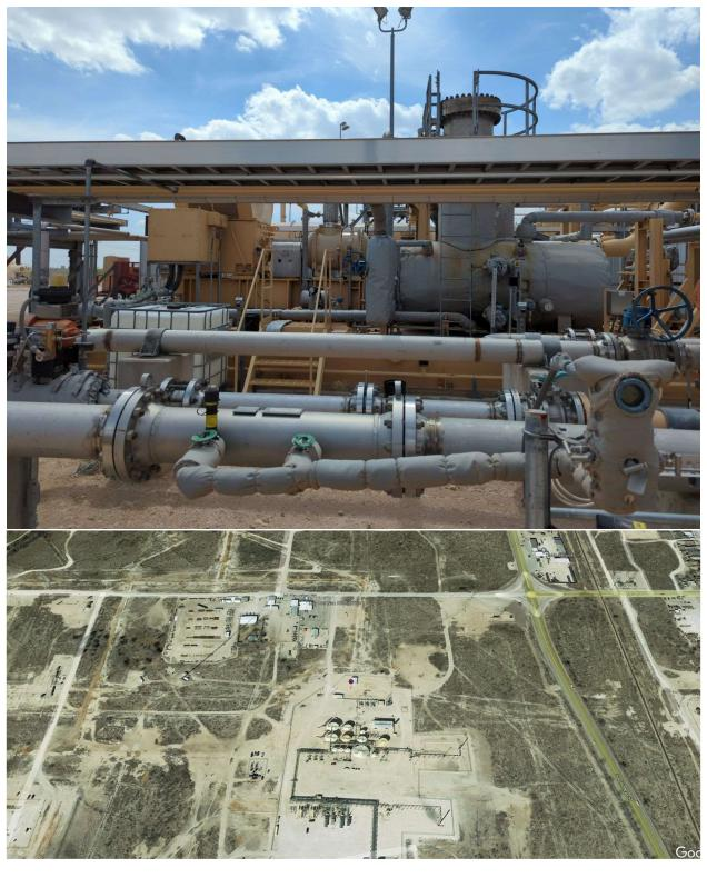
The North Plant had Train A go down. This caused our central tank battery to over pressure and overwhelmed the compressor to the point that it shut down on high high discharge pressure. In order to start the compressor back up we had to get the pressure at the plant back into operating range.
