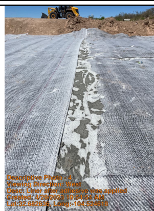
Liner after adhesive was applied
