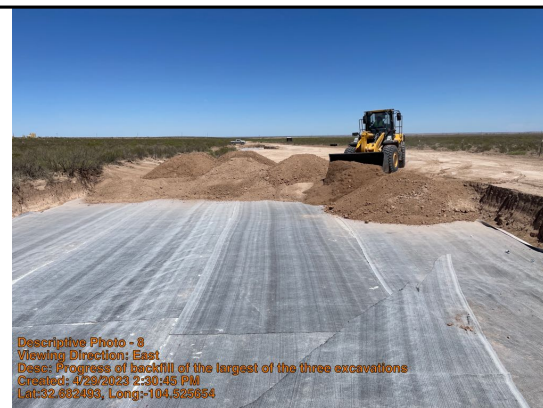
Progress of backfill of the largest of the three excavations
