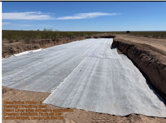
Liner after adhesive application
