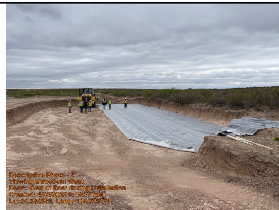
View of liner during installation
