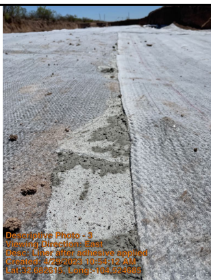
Liner after adhesive applied
