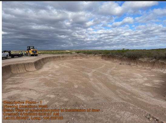
View of excavation prior to installation of liner
