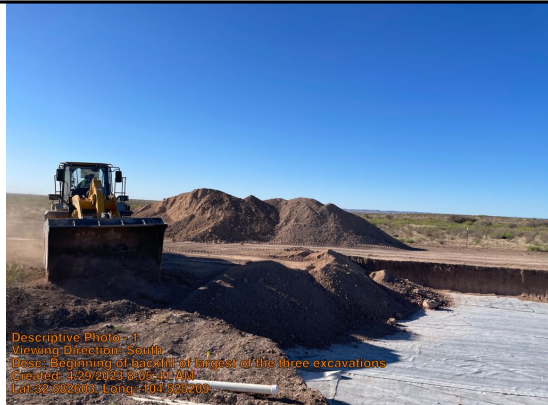
Beginning of backfill of largest of the three excavations
