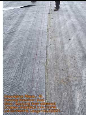
Applying liner adhesive
