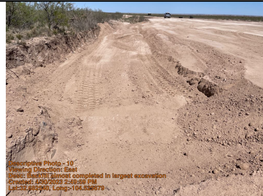
Backfill almost completed in largest excavation
