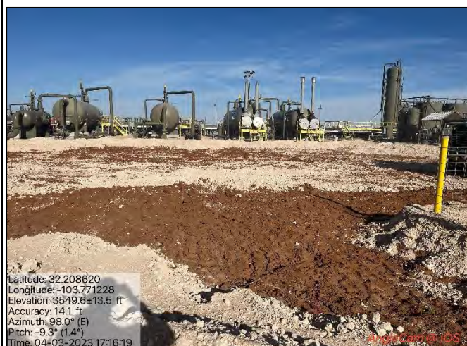
Photograph 3 Date: 04/03/2023 Description: Excavation extent. View: East
