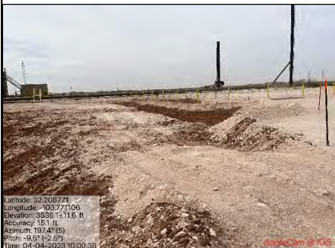
Photograph 4 Date: 04/04/2023 Description: Excavation extent. View: South
