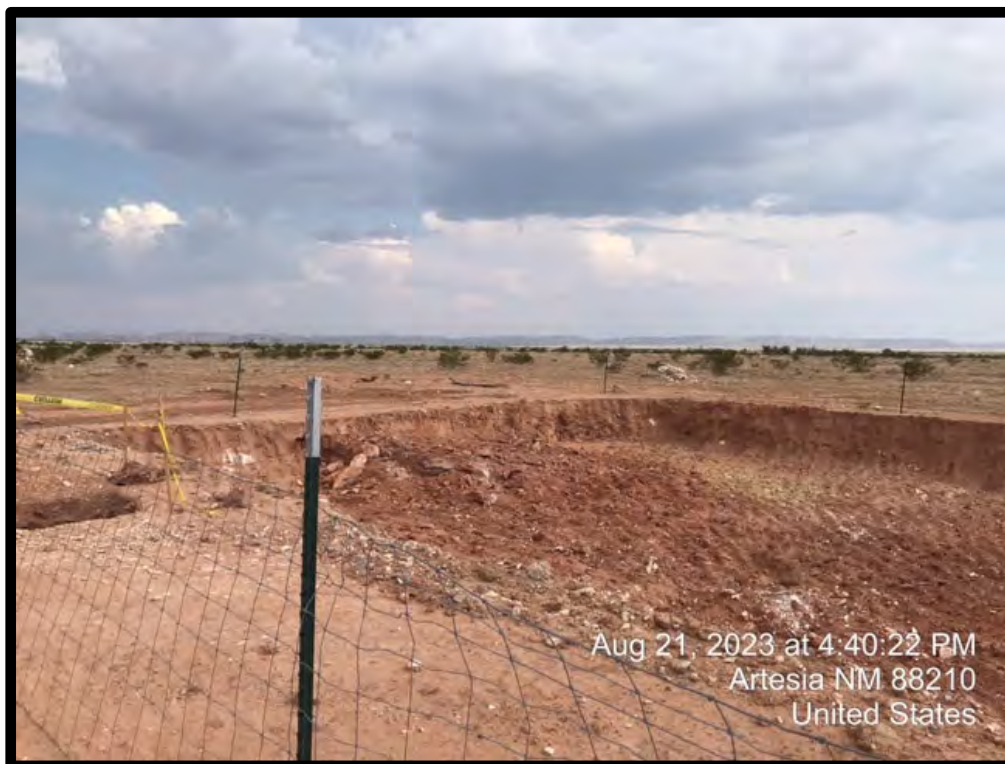
PHOTOGRAPH NO. 2 – A view of the eastern excavation area where due to the encountered lithology, excavation was limited to a depth of one foot below ground surface. The view is towards the southeast.
