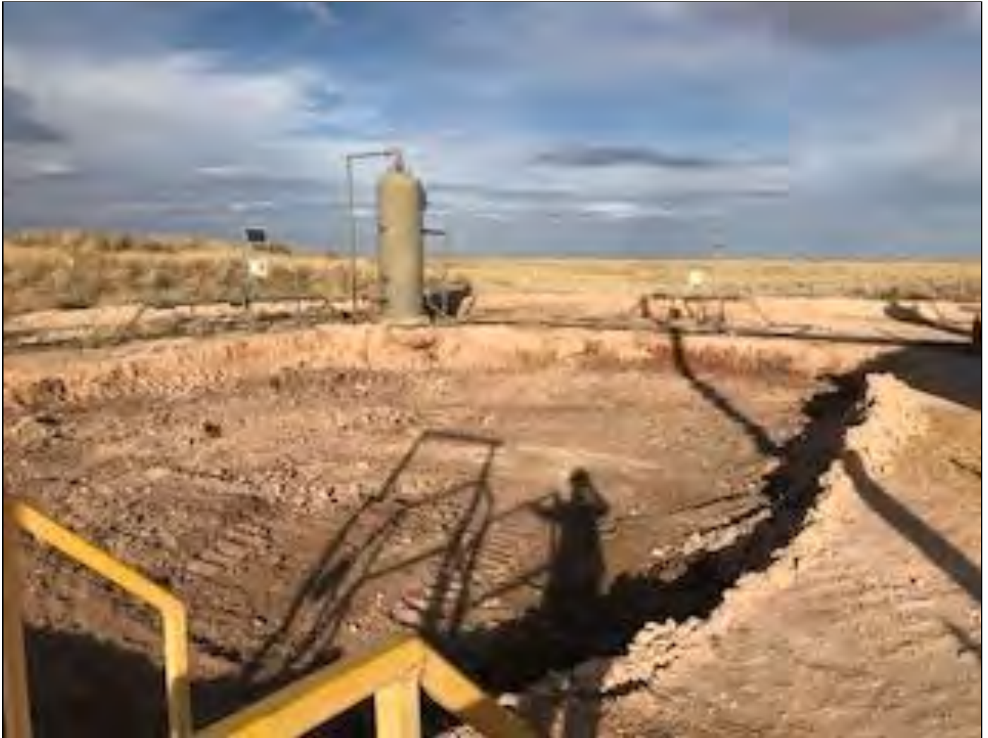
View of excavation facing northeast toward pasture.
