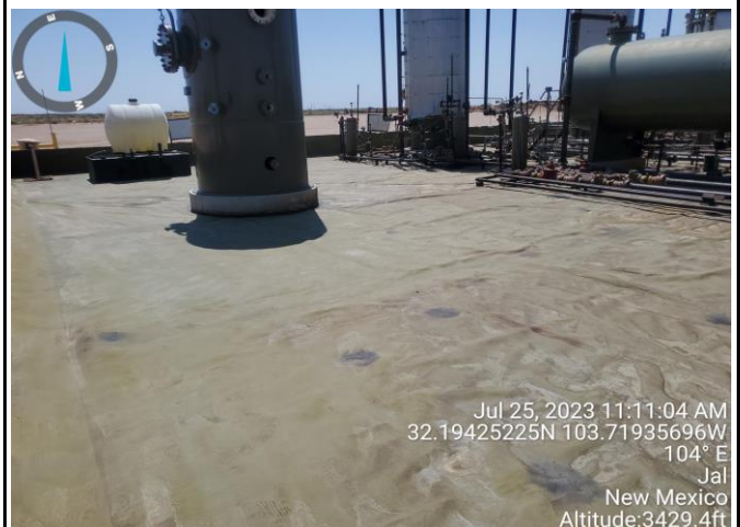
Photograph: 4 Date: 7/25/2023 Description: View of lined containment deemed to be in good condition.
