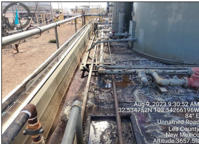
Photograph: 3 Description: View of lined containment deemed to be in good condition View: West
