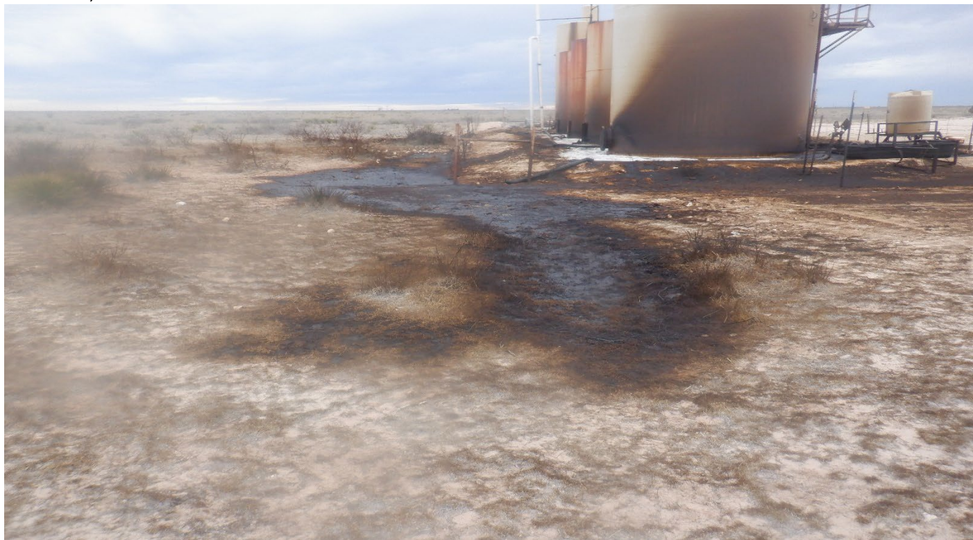
PHOTO #3; LIGHT OIL SPRAY OUTSIDE THE CONTAINMENT AREA:
