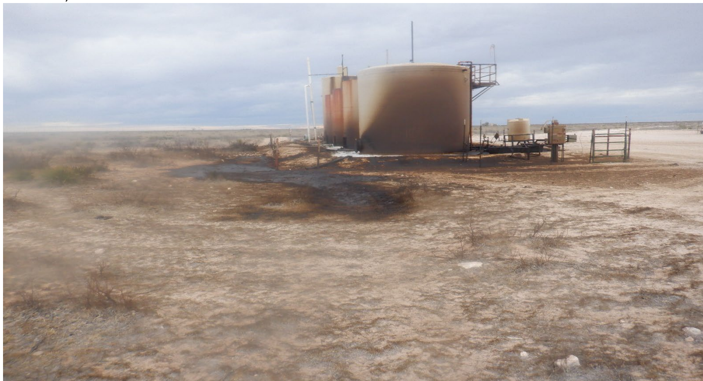
PHOTO #3; LIGHT OIL SPRAY OUTSIDE THE CONTAINMENT AREA:
