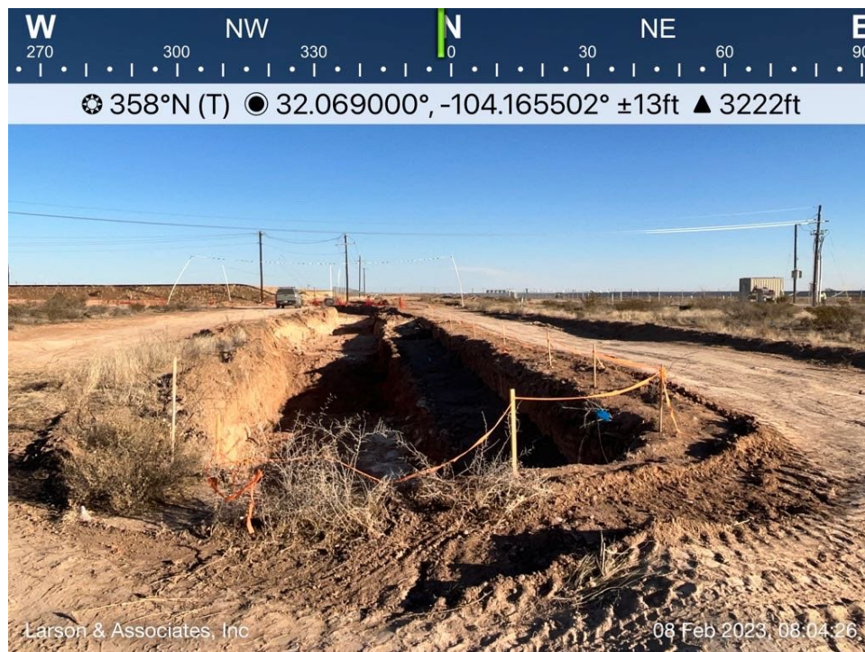
Excavated east area viewing north, February 8, 2023
