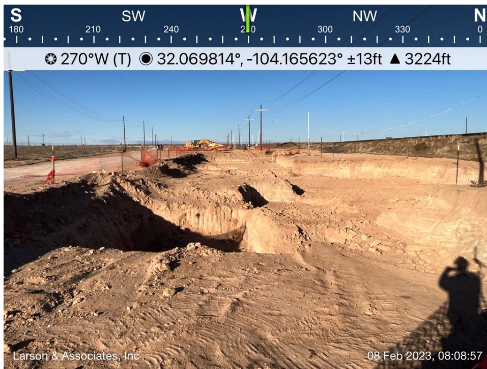
Excavated east area viewing west, February 8, 2023
