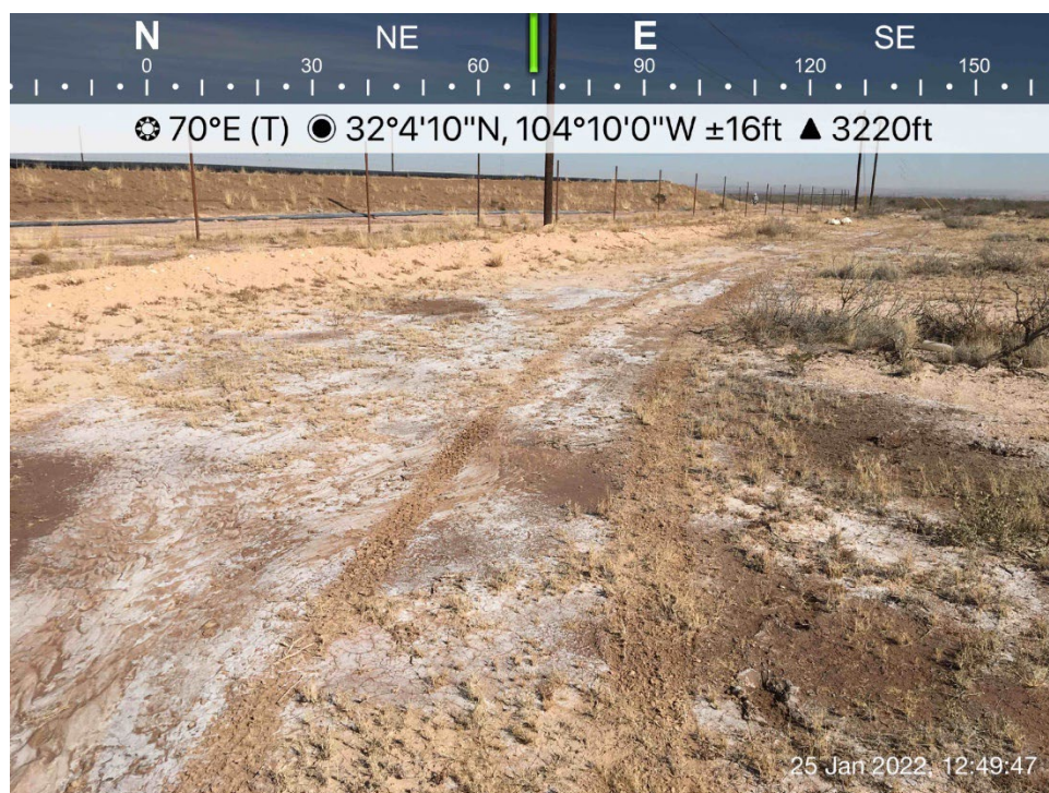
Impacted area viewing east, January 25, 2022
