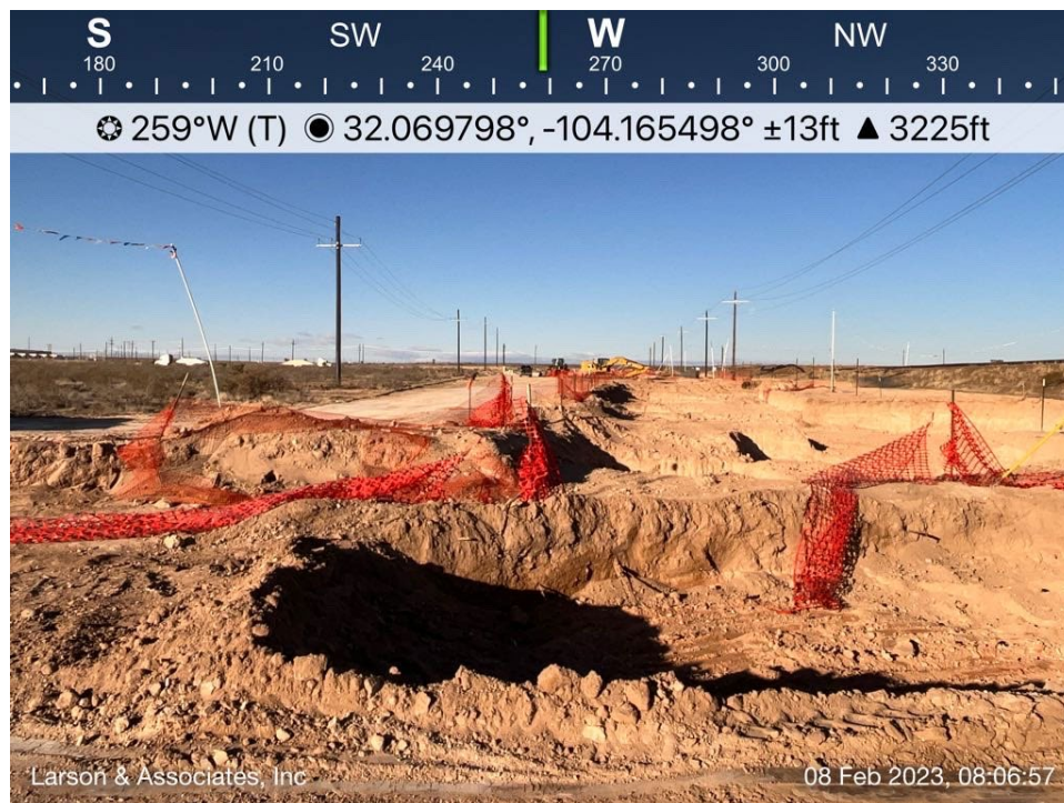
Excavated east area viewing west, February 8, 2023
