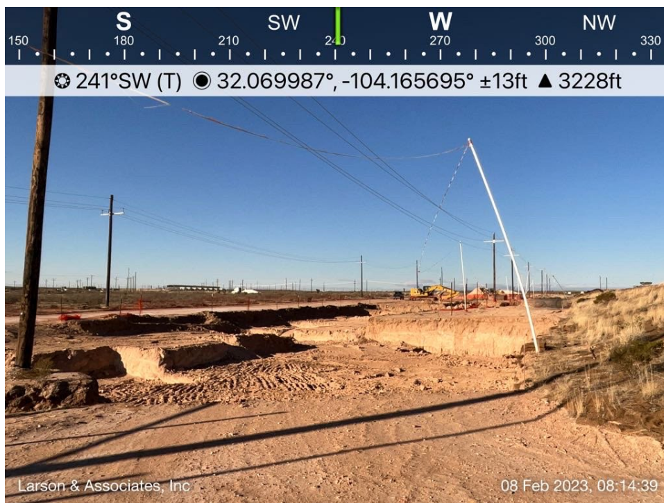
Excavated east area viewing southwest, February 8, 2023
