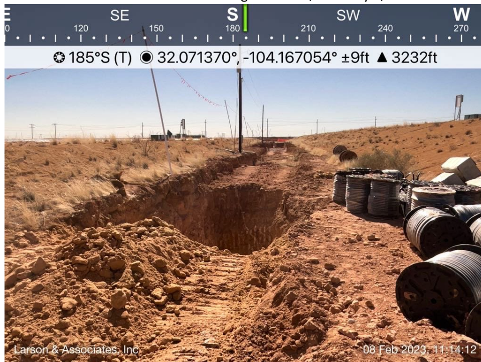
Excavated area viewing south, February 8, 2023
