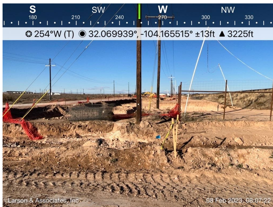
Excavated east area viewing west, February 8, 2023
