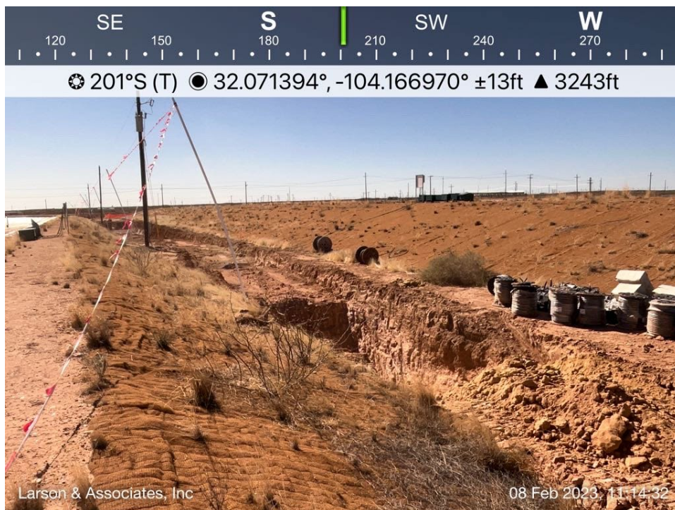
Excavated area viewing south, February 8, 2023
