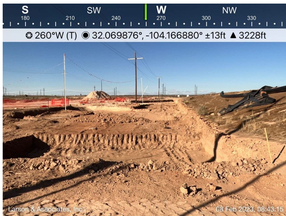
Excavated west area viewing west, February 8, 2023
