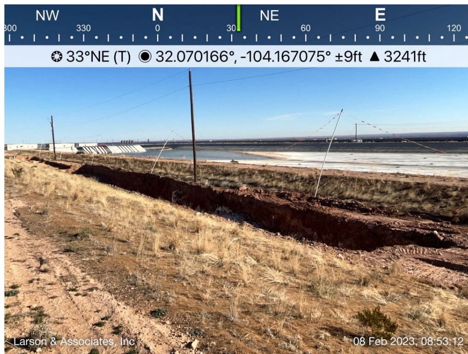
Excavated north area viewing northeast, February 8, 2023
