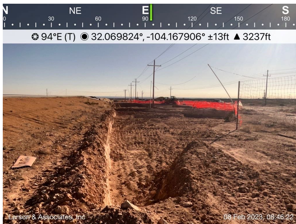
Excavated west area viewing east, February 8, 2023
