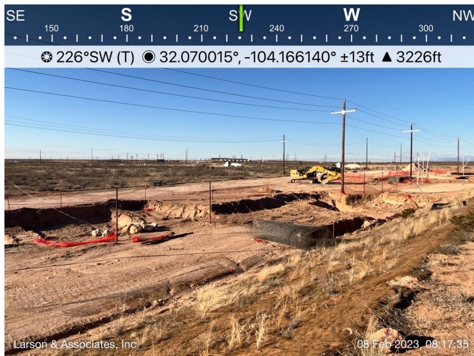
Excavated east area viewing southwest, February 8, 2023
