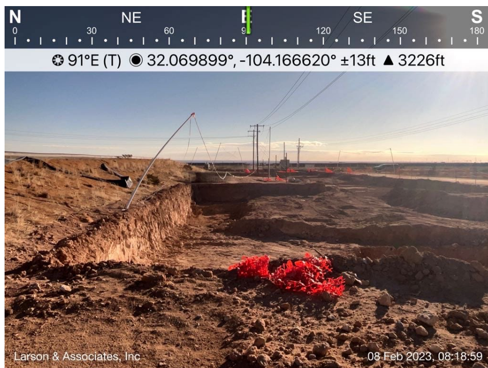
Excavated east area viewing east, February 8, 2023
