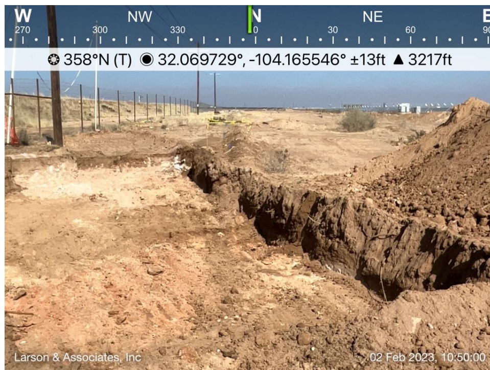
Excavated east area viewing north, February 2, 2023
