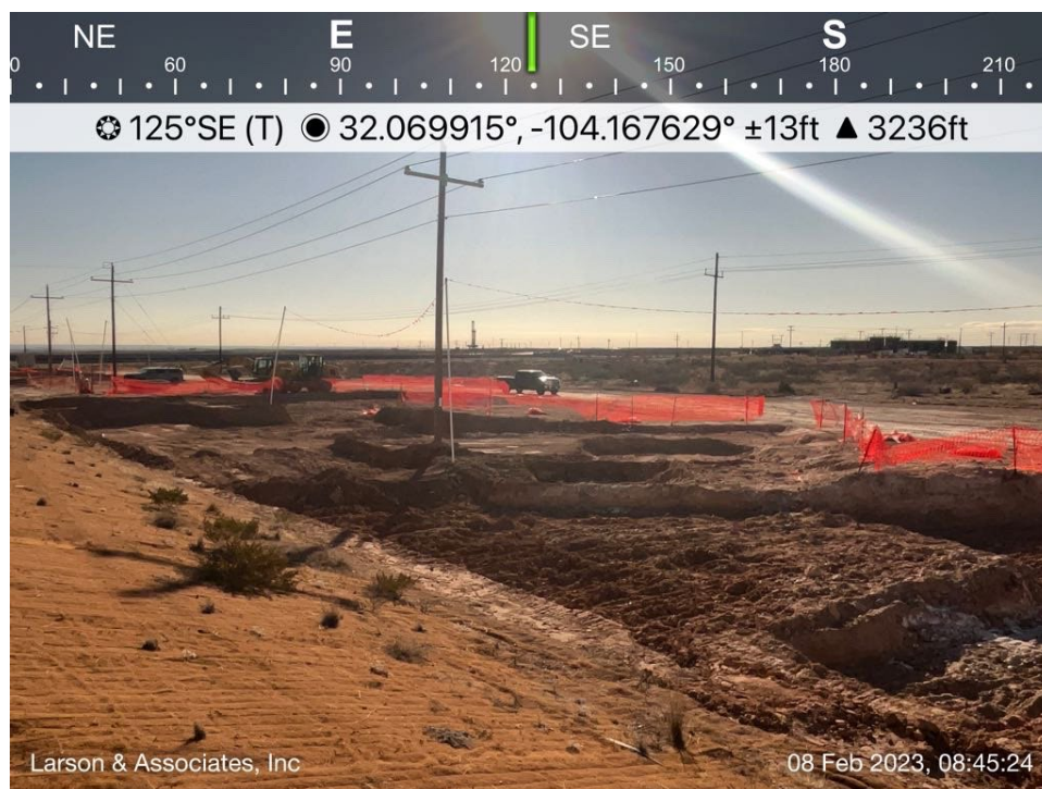
Excavated west area viewing southeast, February 8, 2023
