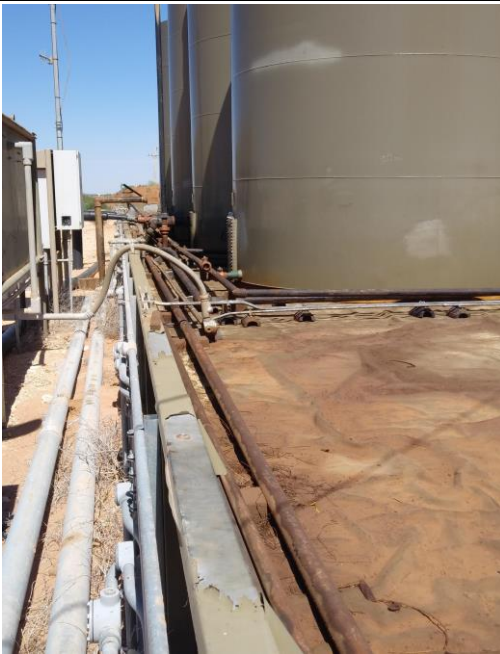
Photograph: 1 Date: 6/19/2023 Description: View of the lined containment deemed to be in good condition, facing east.
