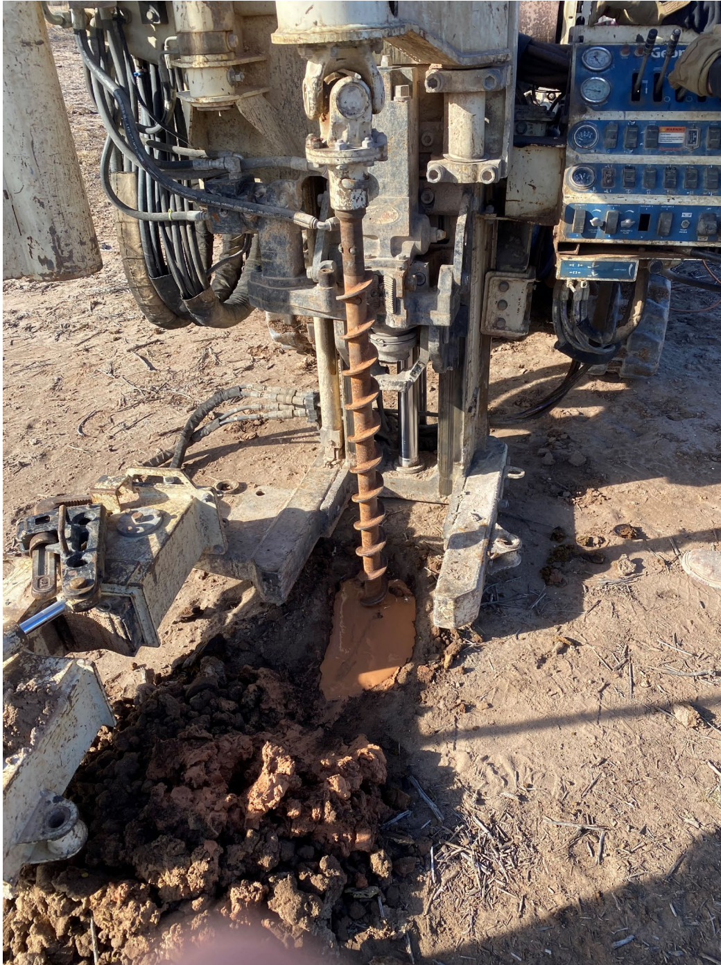
Photo 9: Water zone encountered between 20 and 25 feet below ground surface at 32.562495° -103.996695°.
