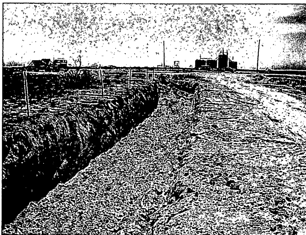
View Southeast – Excavation area of AH-12
