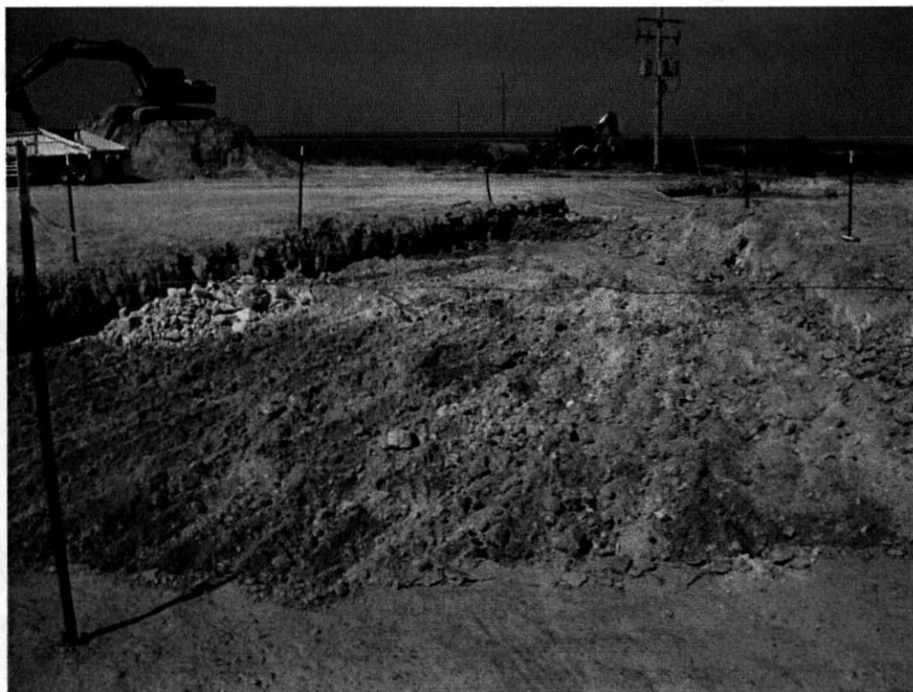
View North – Excavation area of AH-5
