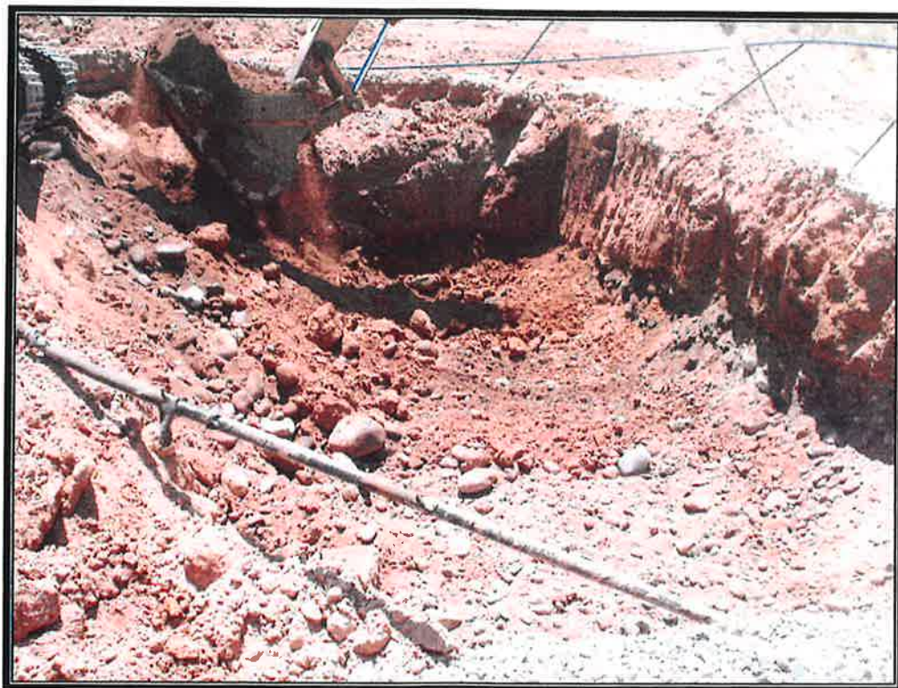
Photo 3: During Excavation with Contaminated Stockpile in Background
