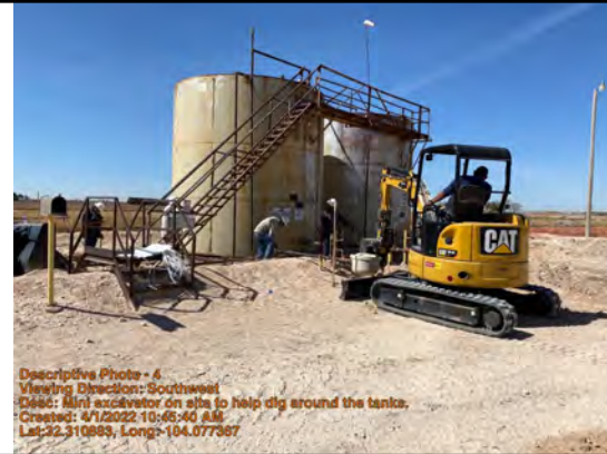
Mini excavator on site to help dig around the tanks.
