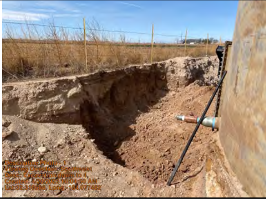
Excavation down to 4'
