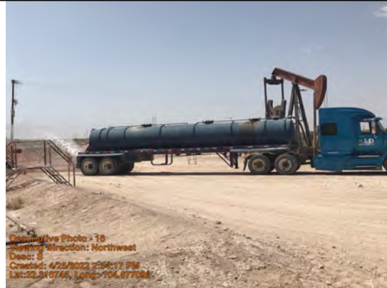
LD Construction Tanker Truck dumping fresh water on Caliche for packing
