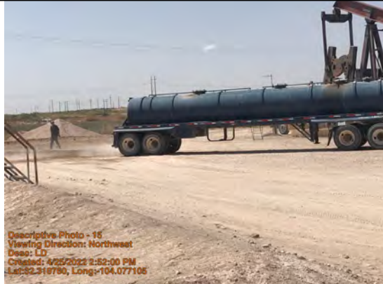
LD Construction Tanker Truck dumping fresh water on Caliche for packing
