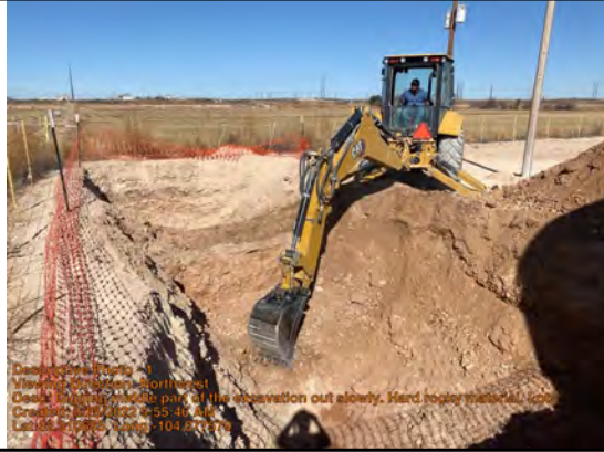
Digging middle part of the excavation out slowly. Hard rocky material. Lots of river rock
