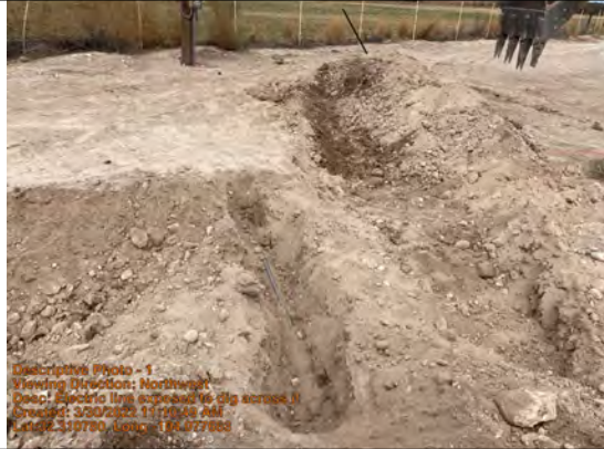
Electric line exposed to dig across it
