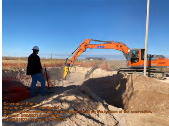
Jackhammer breaking the hard material on the bottom of the excavation.
