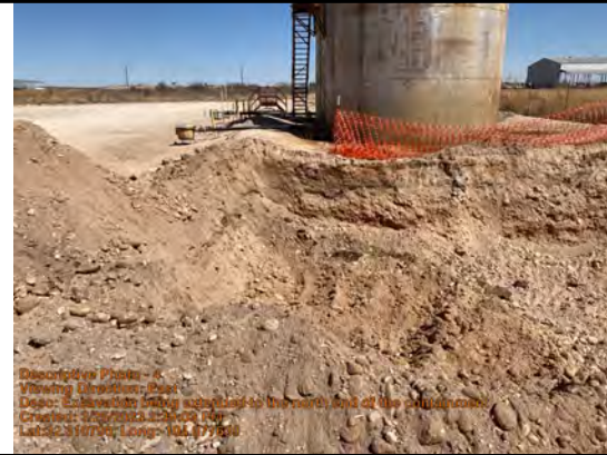
Excavation being extended to the north end of the containment
