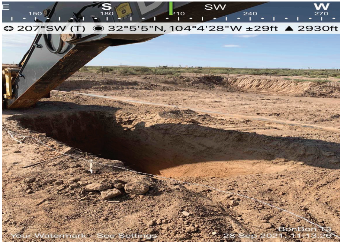
View of Remediation Activities – View South
