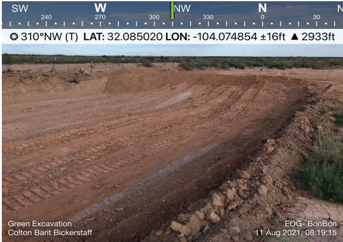
View of Remediation Activities – View West
