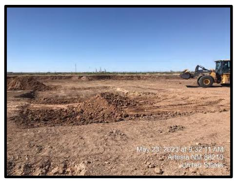
PHOTOGRAPH NO. 3 – A view of over-excavation activities in areas documented to have elevated TPH concentrations. The view is towards the south.
