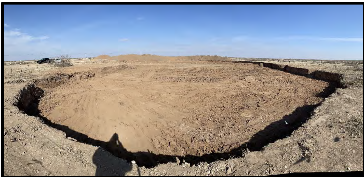
PHOTOGRAPH NO. 3 – An additional view of excavated area upon completion of the soil removal operations. The material designated for re-use can be seen in the background of the photograph. The view is towards the east.
