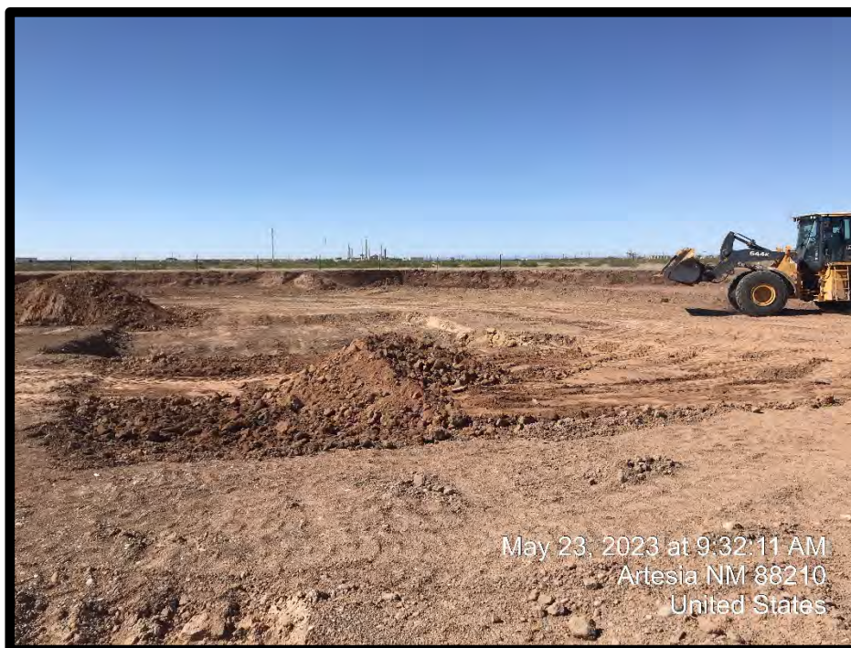
PHOTOGRAPH NO. 3 – A view of over-excavation activities in areas documented to have elevated TPH concentrations. The view is towards the south. (Approximate GPS: 32.724539, -104.442978)
