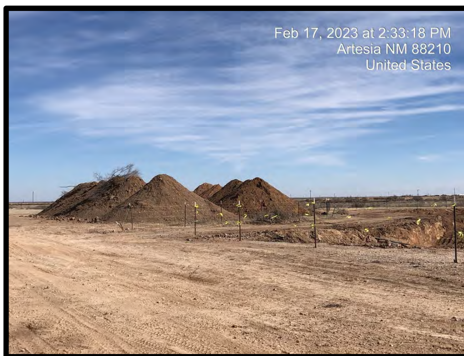
PHOTOGRAPH NO. 2 – A view of stockpiled material awaiting assessment sampling to determine if the material was suitable for re-use. The view is towards the southeast.
