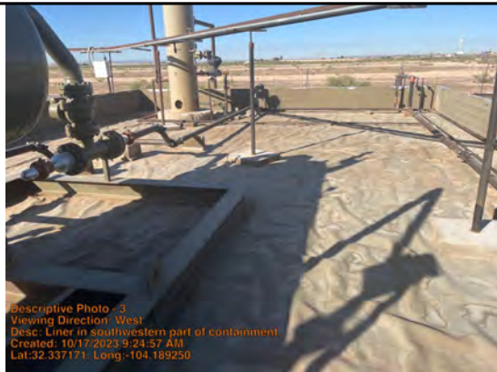
Liner in southwestern part of containment.
