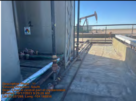
Liner in central part of containment.
