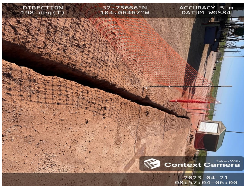
PHOTO 3: View of the hydro-vac spotting of lines.
