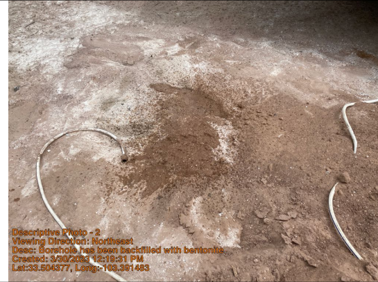
Borehole has been backfilled with bentonite
