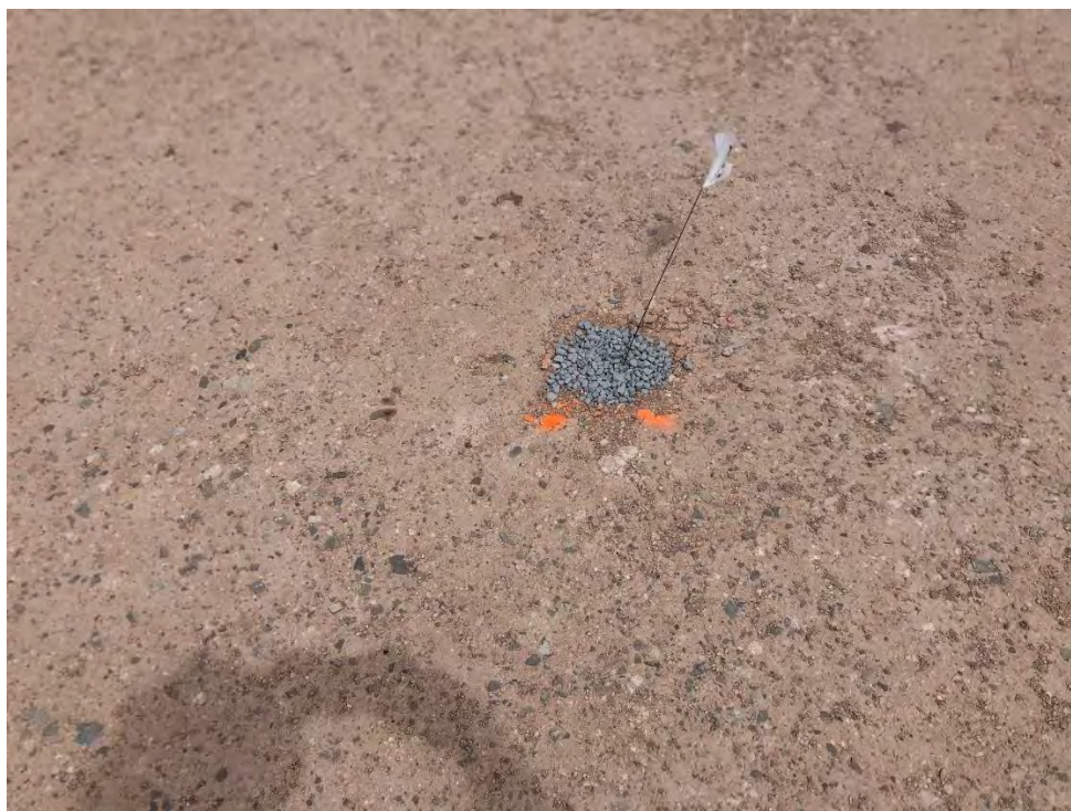
Photo 7. View of a borehole filled with bentonite
