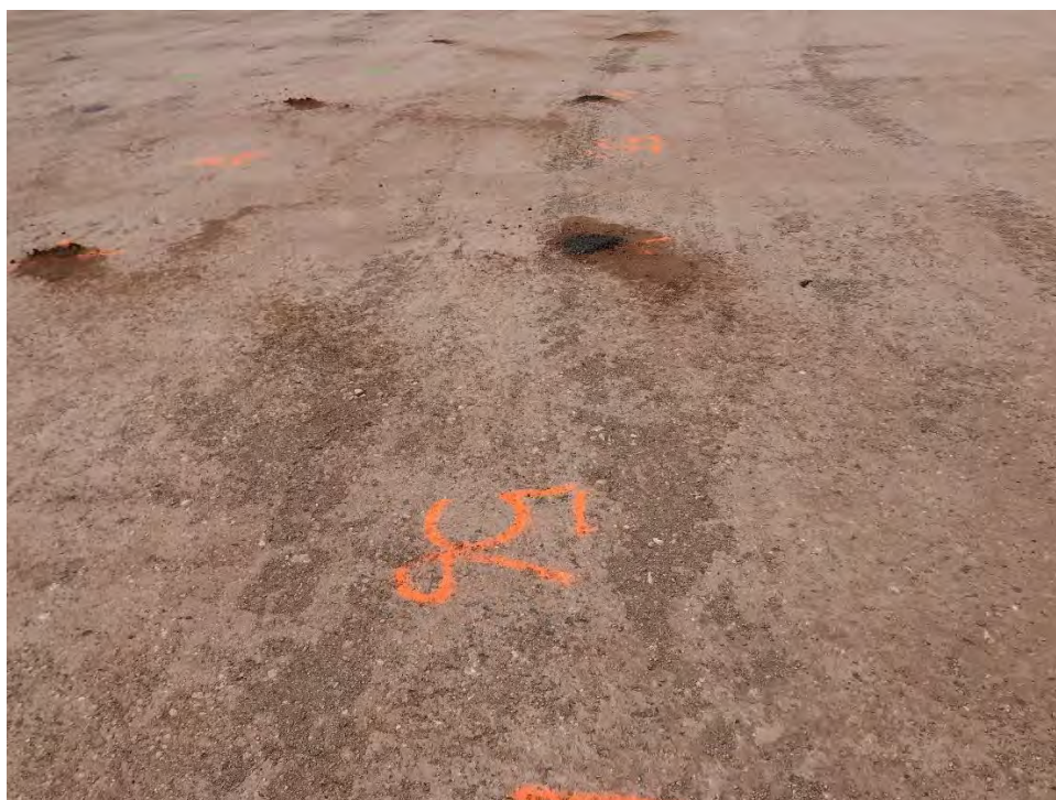
Photo 8. View to the west of boreholes filled with bentonite and hydrated to ensure an effective seal
