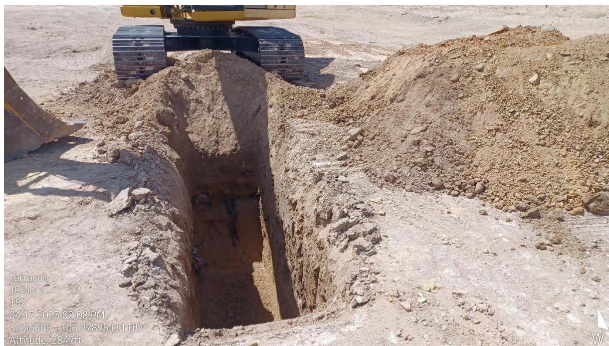
PHOTO 6: View of the sample location 182, with liner exposed in the sidewall
