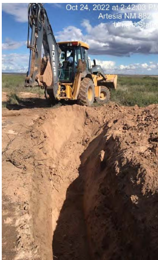
PHOTOGRAPH NO. 4 – A typical view of the vertical delineation test trench sampling activities conducted on October 24, 2022.
