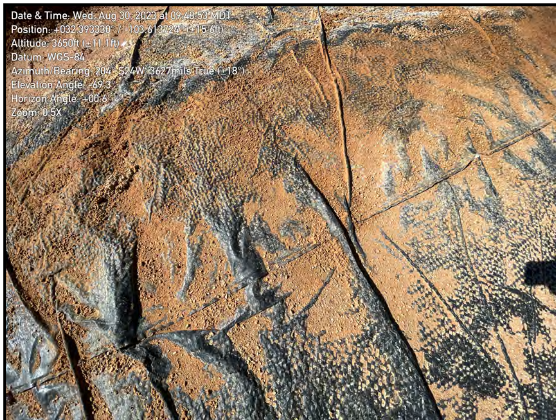
View of newly installed liner on eastern portion of tank battery.
