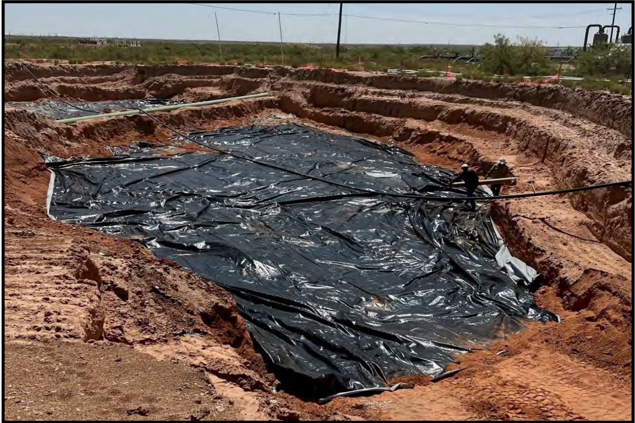
View of liner placed in excavation area prior to backfill, facing southeast.
