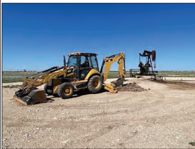
Photograph: 2 Date: 9/6/2022 Description: Delineation activities View: Southwest
