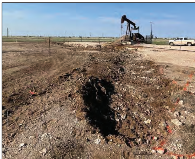
Photograph: 4 Date: 9/30/2022 Description: Excavation activities View: Southwest
