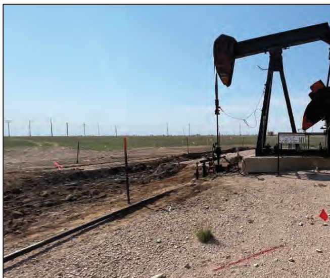
Photograph: 3 Date: 9/30/2022 Description: Excavation activities View: Southeast
