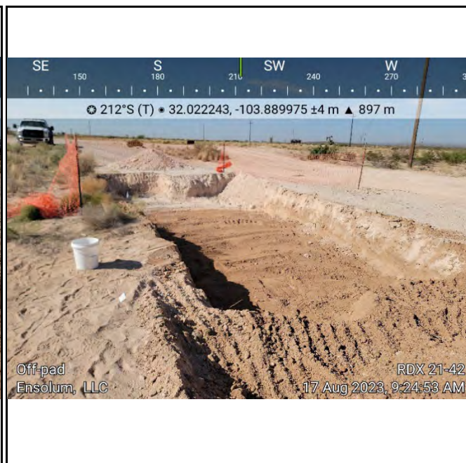
Photograph 4 Date: 8/17/2023 Description: Partial backfill to allow truck access. View: Southwest
