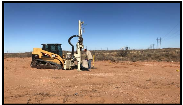
View of soil boring (SB-1) installation near release point on Enterprise Trunk A pipeline, facing northwest.
