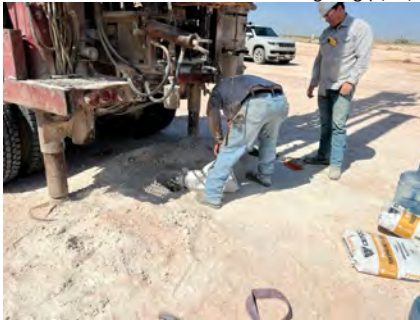
View to SW of plugging boring BH-1 (7/19/22).
