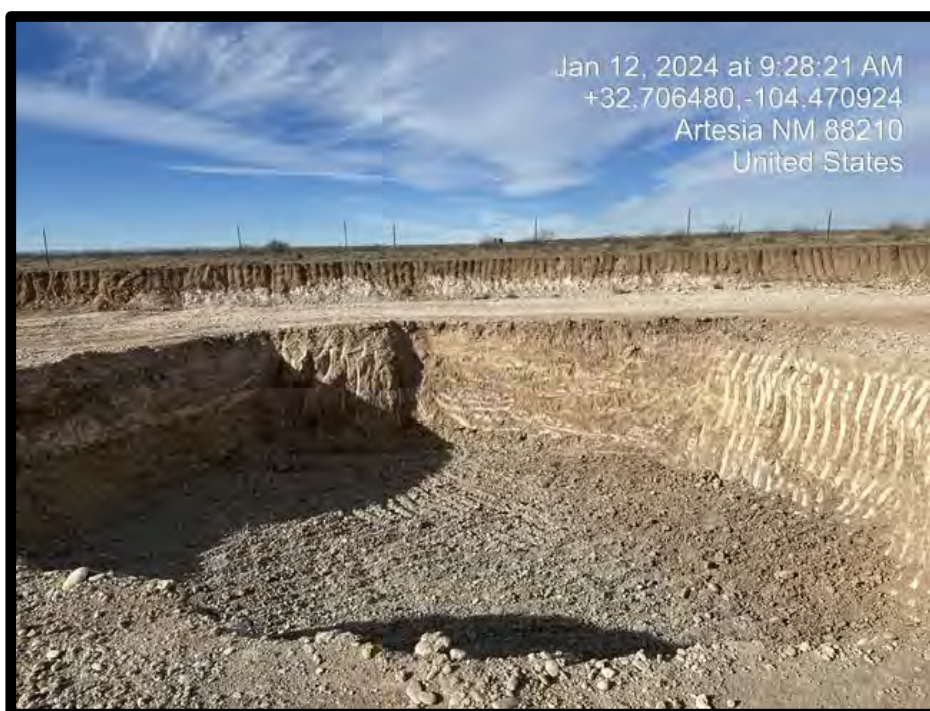
PHOTOGRAPH NO. 9 – An additional view of the area excavated to a depth of approximately 13 feet bgs upon completion of the removal process. The view is towards the west.
