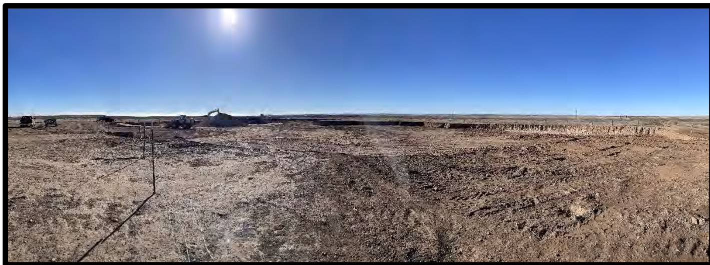
PHOTOGRAPH NO. 7 – A view of primary excavation area (Area A) upon completion of the removal activities to four feet bgs. The view is towards the south. (Approximate GPS: 32.706480, -104.470374)
