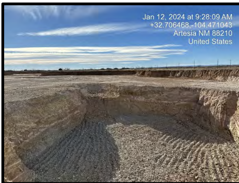
PHOTOGRAPH NO. 9 – A view of the area excavated to a depth of approximately 13 feet bgs upon completion of the removal process. The view is towards the south.
