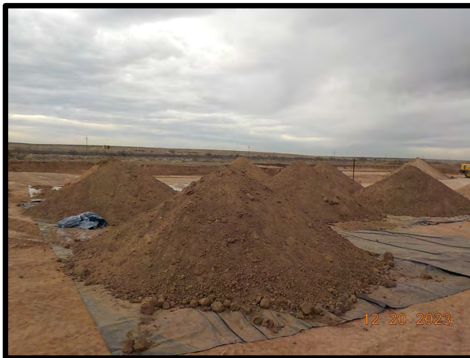
PHOTOGRAPH NO. 3 – A view of the material for potential re-use, segregated in approximate 100 cubic yard stockpiles and on plastic liner. The view is towards the northwest.
