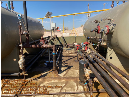
Liner between the north separators
