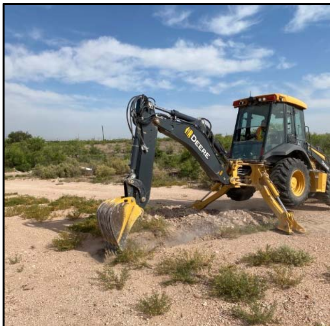
Photo 7: Advancing test pit at sample location B08. Direction: Northeast
