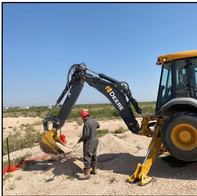
Photo 5: Advancing test pit at sample location B05. Direction: Northwest
