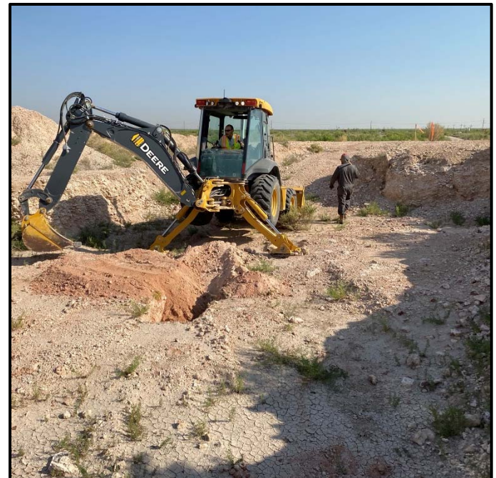
Photo 4: Advancing test pit at sample location B03. Note: Location is inside former pit, which is below the natural ground surface. Direction: Southeast
