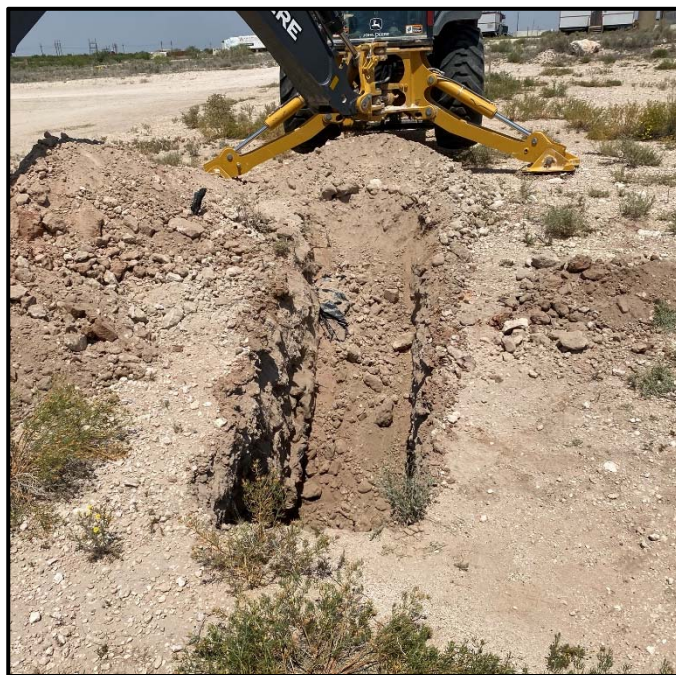
Photo 6: Advancing test pit at sample location B07. Direction: South (down)
