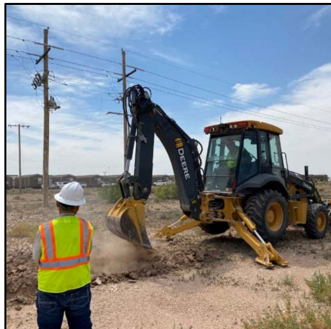
Photo 8: Backfilling the test pit at sample location B11 after sample collections and field measurements were performed. Direction: East-Southeast
