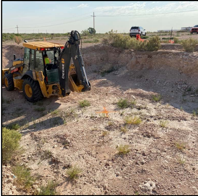
Photo 1: Setting up backhoe before advancing test pit at sample location B03. Note: Location is inside former pit, which is below the natural ground surface. Direction: Northeast
