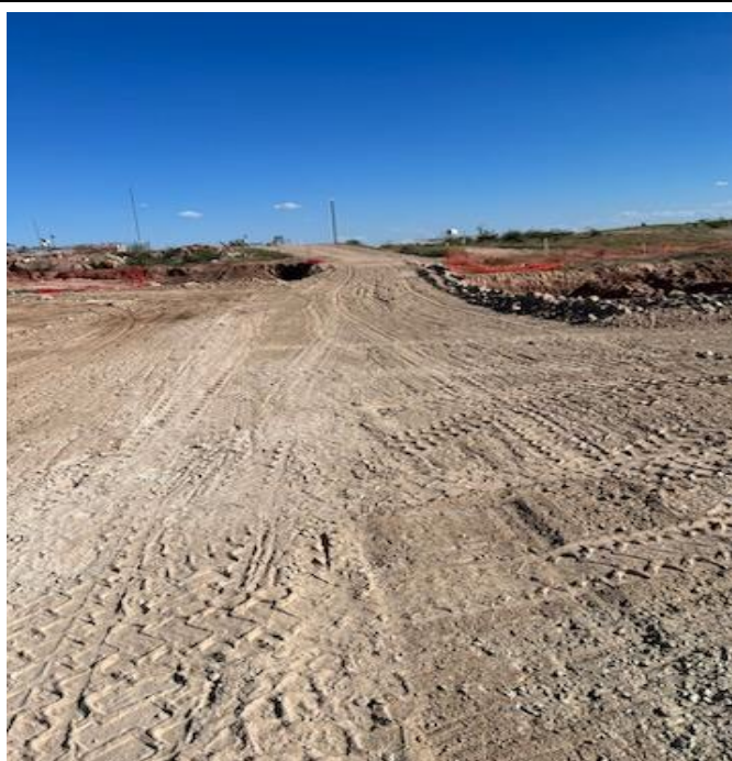
Backfill to grade lease road.
