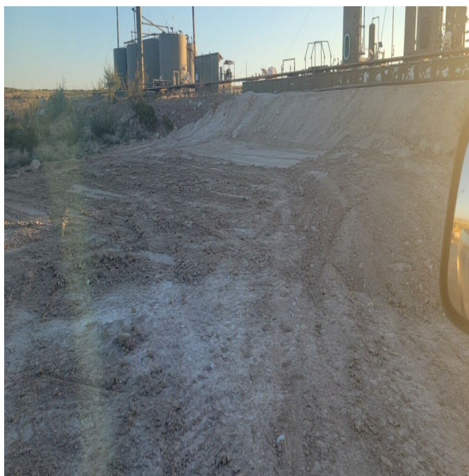
Pad Area Backfilled to Grade
