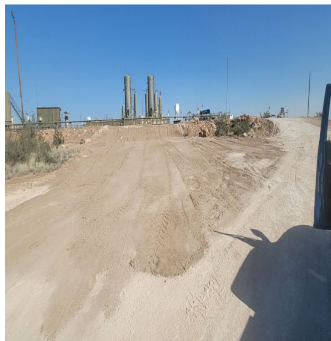
Pasture Backfilled with Topsoil
