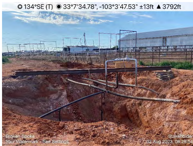
Photo #14 - Photo view of release area after further excavation of impacted soils (02Aug23)
