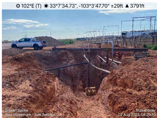
Photo #15 - Photo view of release area after further excavation of impacted soils (02Aug23)
