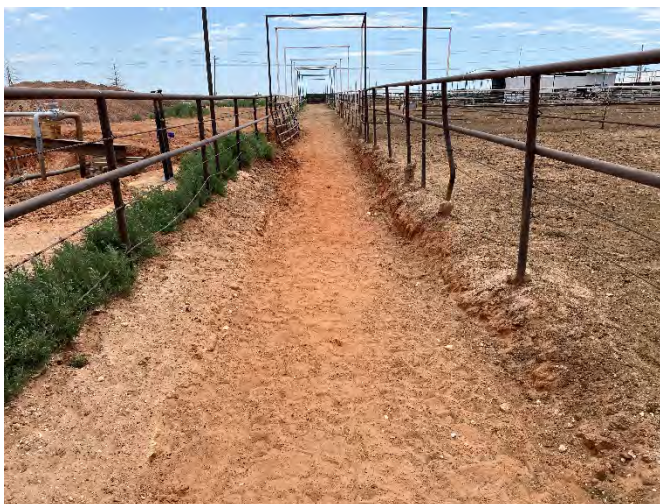
Photo #18 - Photo view of release area after further excavation of impacted soils (02Aug23)
