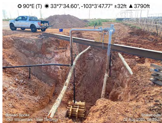
Photo #16 – Photo view of release area after further excavation of impacted soils (02Aug23)
