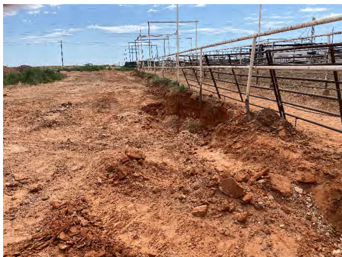
Photo #17 – Photo view of release area after further excavation of impacted soils (02Aug23)
