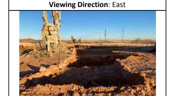
Southwest of pump jack facing east. Scrape to 1 foot bgs on west side completed.
