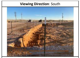
Northeast edge of excavation facing south. Excavation to 4 feet bgs completed.
