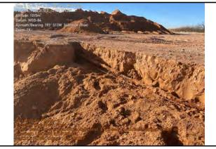
South of artificial lift facing west. Exposed conduit collapsed under its own weight.
