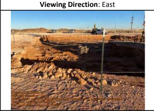
North of pump jack facing east. Excavation to 4 feet bgs completed.
