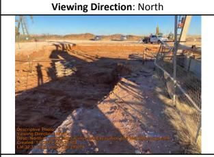
North of pump jack facing east. Excavation to 4 feet bgs completed.
