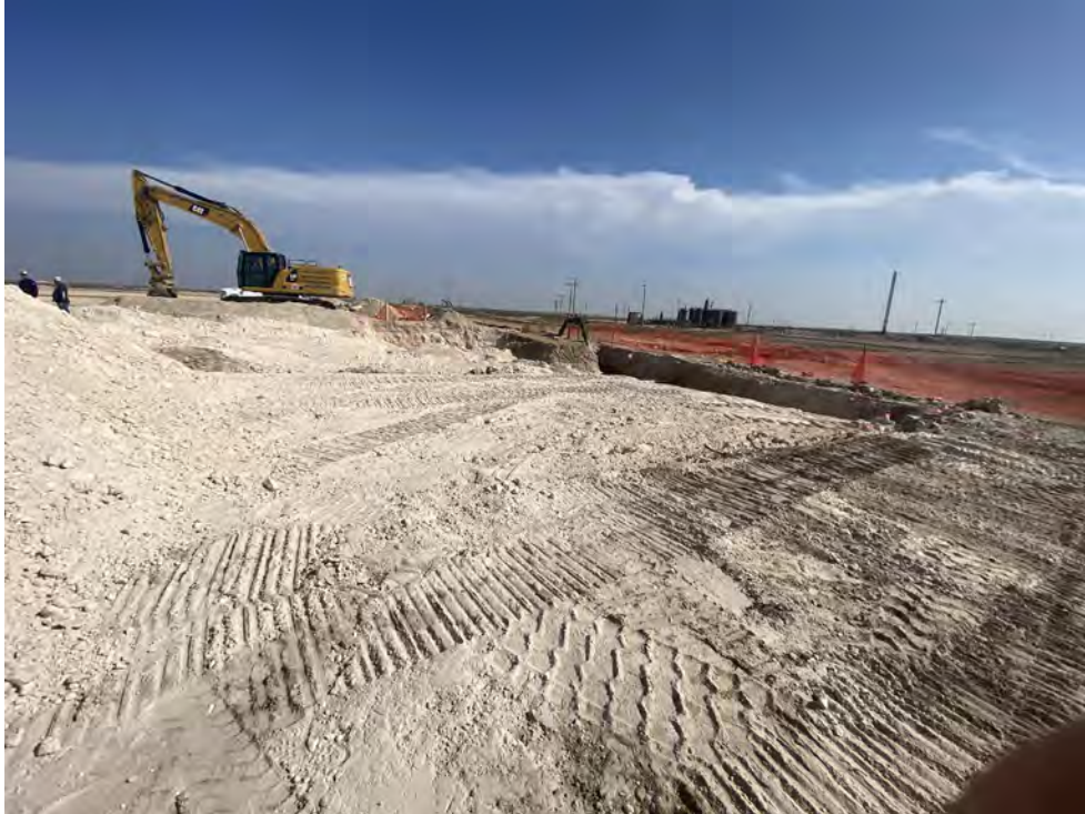
View showing backfill of excavation area
