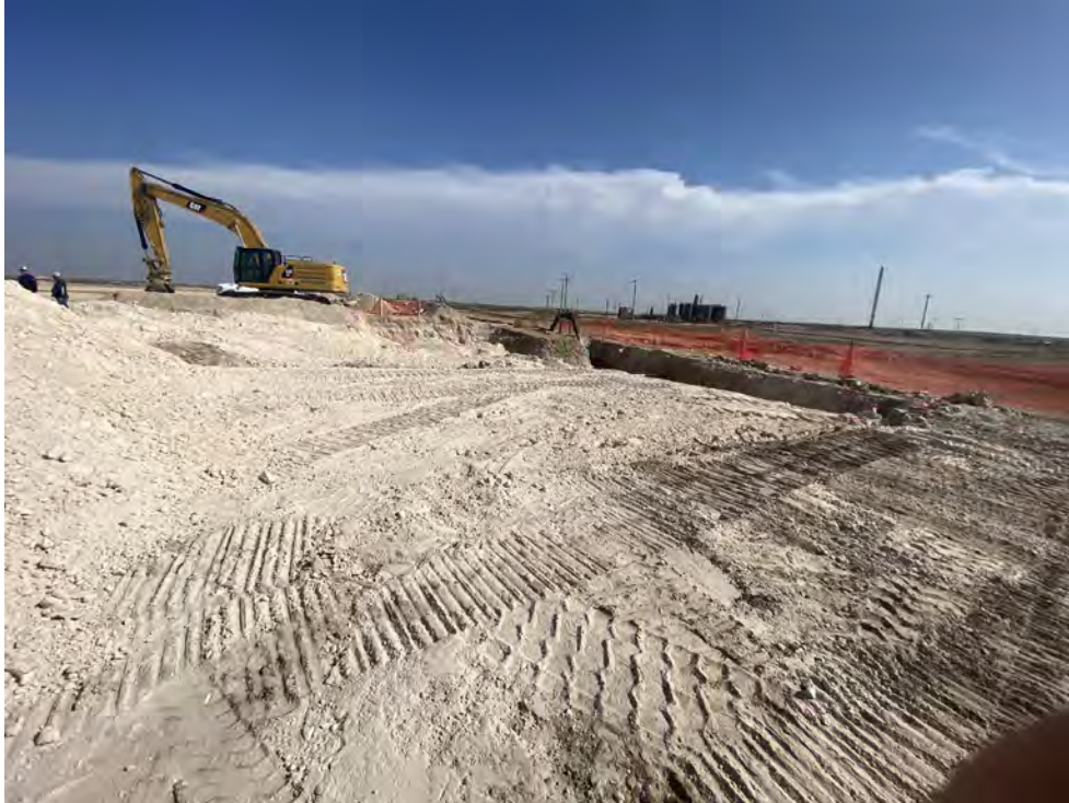
View showing backfill of excavation area
