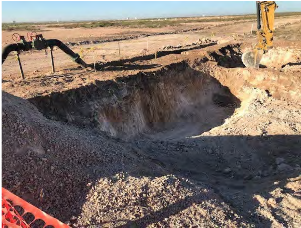
View of active soil remediation south of point of release immediately adjacent to pipeline
