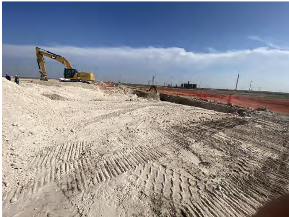
View showing backfill of excavation area
