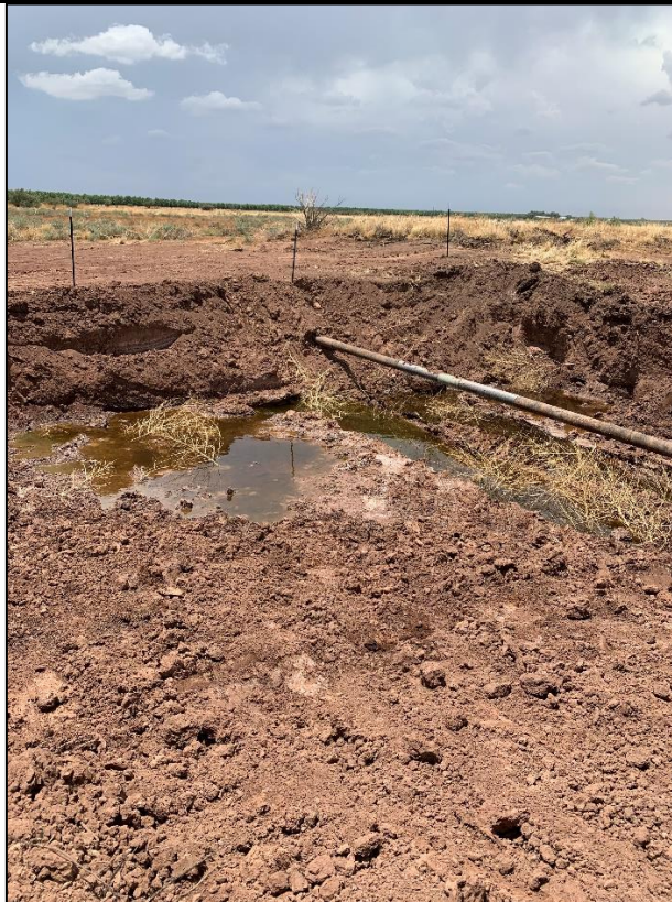
PHOTO 4: View of final Excavation, after trench dewatering and pipe repair.
