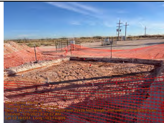
Excavation at 1 foot depth and 25x26 feet length and width with plotted sampling points with white flagging
