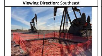
Excavation at 1 foot depth and 25x26 feet length and width with plotted sampling points with white flagging
