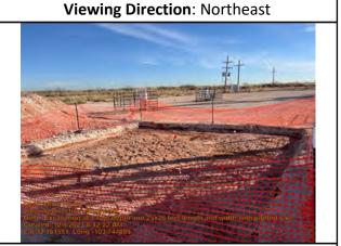
Excavation at 1 foot depth and 25x26 feet length and width with plotted sampling points with white flagging
